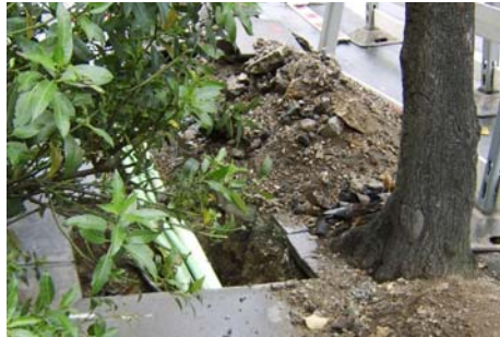
Utility works near a tree
