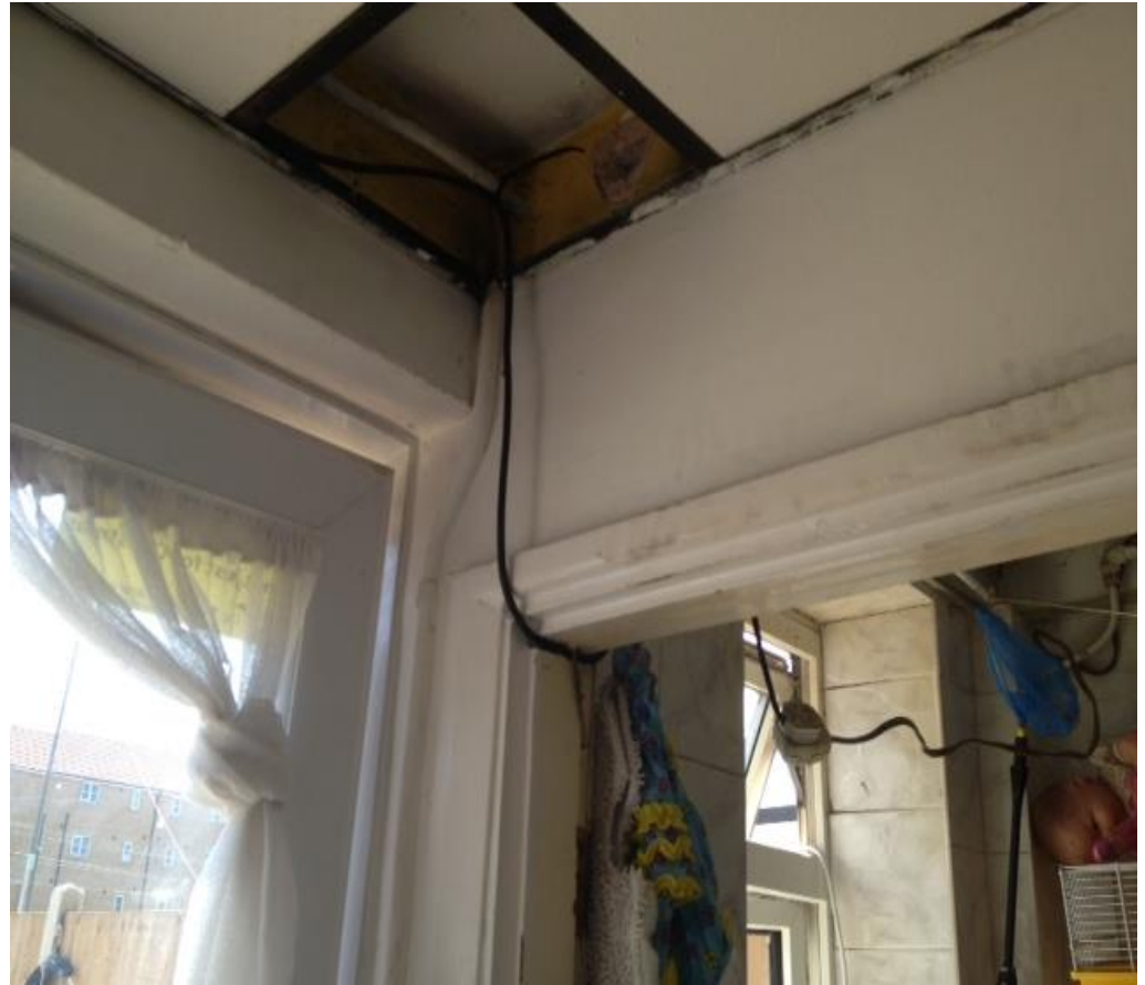
Trailing electrical leads
