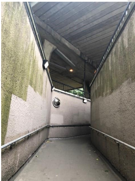
Image 1: Subway under the Croydon Flyover – the only pedestrian route through Old Town Roundabout
