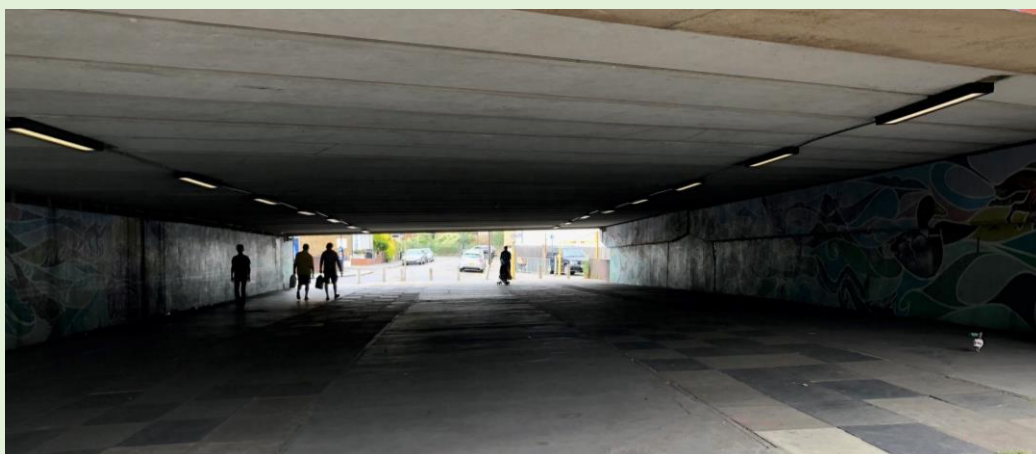
Pedestrian underpass at Reeves Corner
