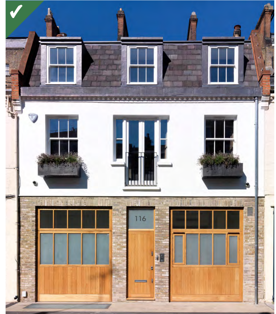
Figure 4.20d: The addition of 3 dormers that have been sympathetically designed to the existing building and respond to the positioning of the windows below.
