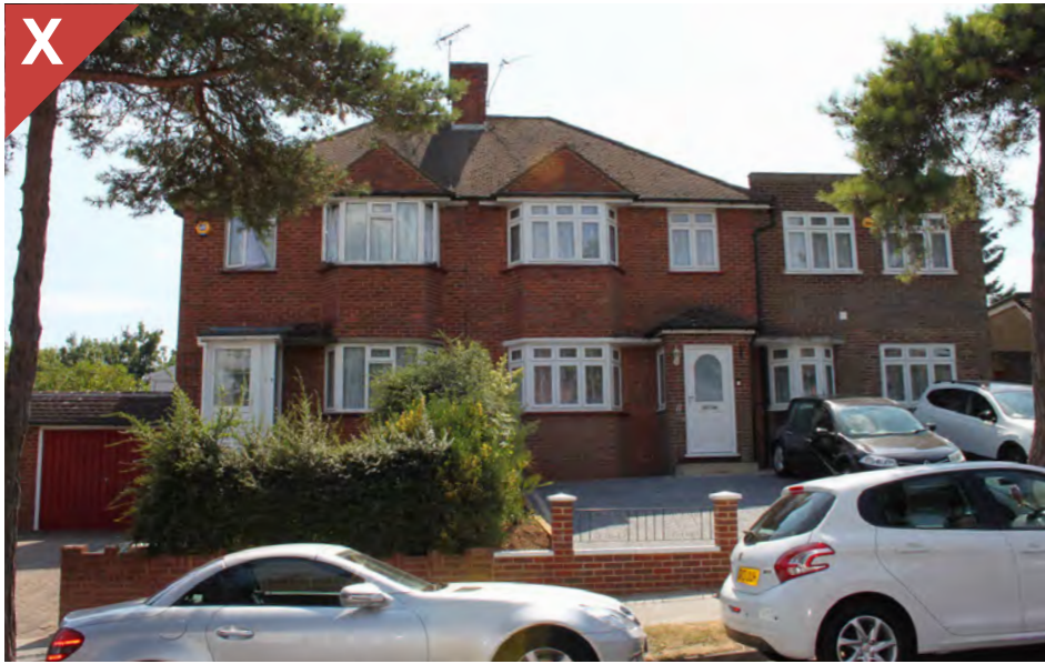
Figure 4.16b: A low-quality two storey side extension which is overly dominant, upsetting the balance of this pair of semi-detached homes. The brick neither match nor distinguish from the existing and the junction at the eaves is poorly detailed.
