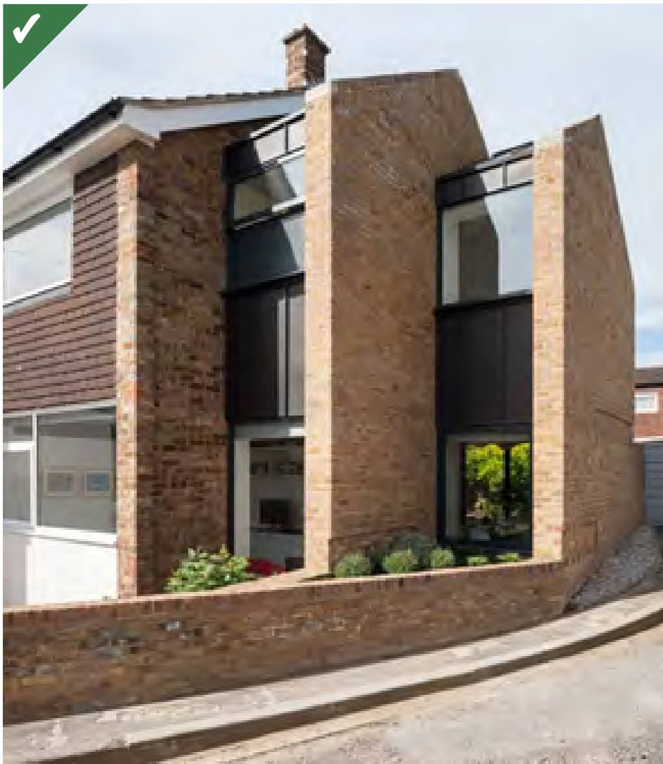
Figure 4.16c: Example of a subservient two-storey side extension that introduces contemporary elements, such as the windows and their surrounds, to help distinguish the new from the existing.
