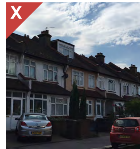
Figure 4.20e: Example of where a side roof extension has not been setback from the original roof, compromising the composition of the original house.
