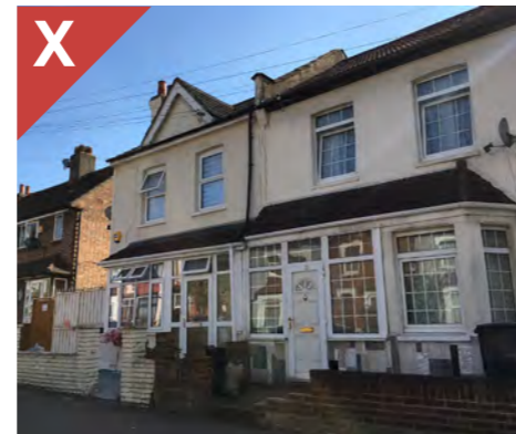
Figure 4.4h: A poor example of two porches that have been built up to and over original bay windows. The design fails to respond to the historic pattern of development and materials are low quality.
