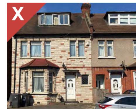
Figure 4.9g: An example of inappropriate cladding to a house that hinders the appearance of the street.
