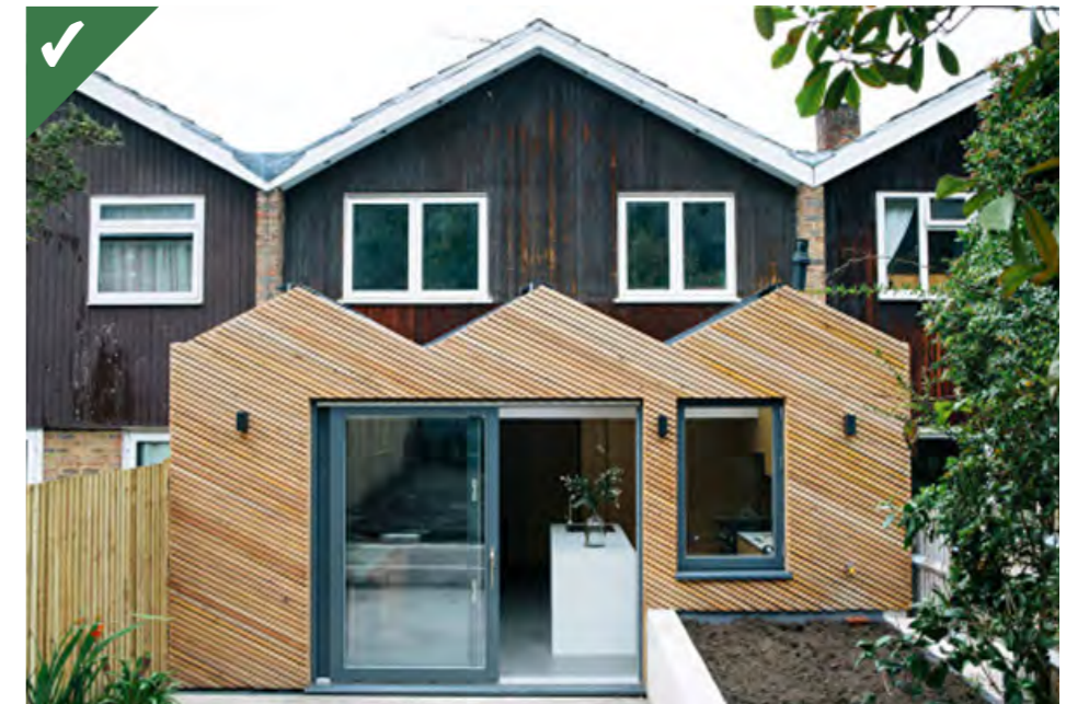
Figure 4.14a: An example of a roof design to a single storey extension that has been designed to ensure it doesn't overlap with the windows above.
