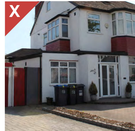
Figure 4.11b: A poorly designed single storey side extension that fails to respond to the original dwelling. It has an awkward combination of roof forms and the appearance is further exacerbated by the porch extension, which hasn't been combined with the side extension.
