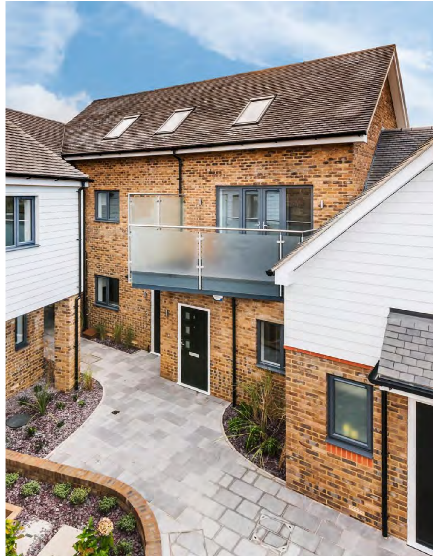
Figure 2.4.1m: Overlooking is minimised through careful orientation of built form and the use of screening to balconies. This scheme may have been improved by the use of perforated screening to the balcony, rather than frosted glass.
