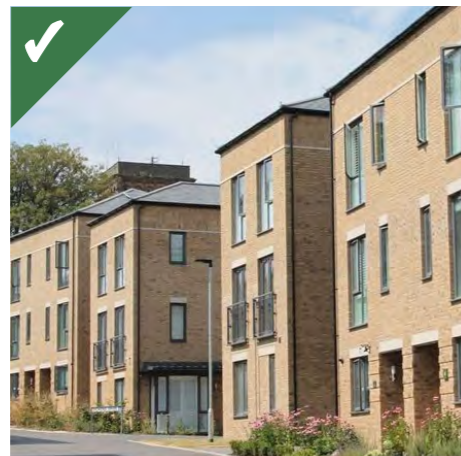
Figure 2.5.6c: Example of where placement of servicing items has been considered early in the design development, ensuring elevations are kept free of clutter
