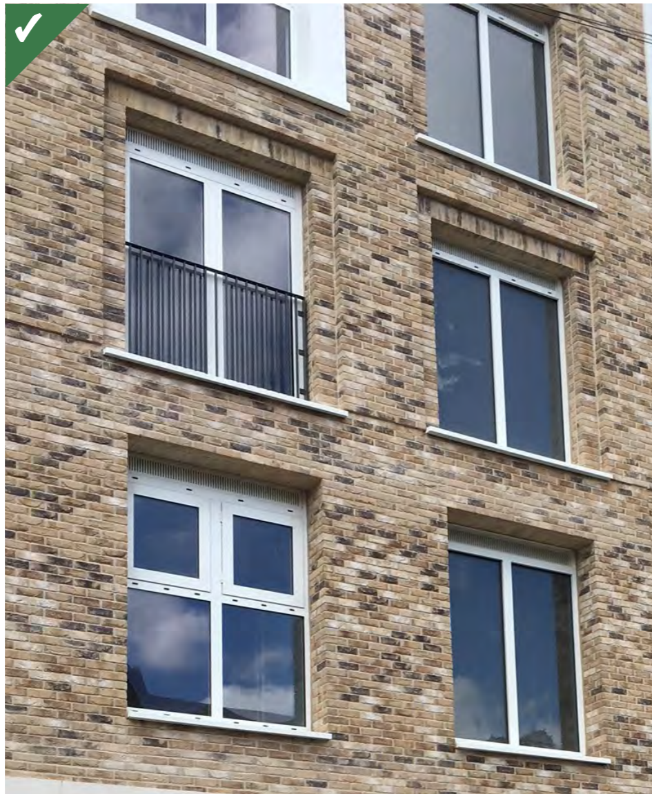
Figure 2.5.4a: Deep reveals provide a sense of solidness that can add appeal to facades. Varied depths of reveals adds interest to the facade.
