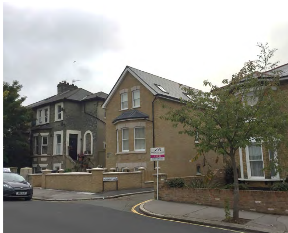
Figure 1.4b: A development of new flats in the East India Conservation Area
