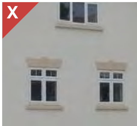
Figure 2.5.4b: Shallow reveals can result in a poor appearance that lacks depth and windows appear as if they are stuck on. Shallow reveals should generally only be used where they are part of a compelling design.
