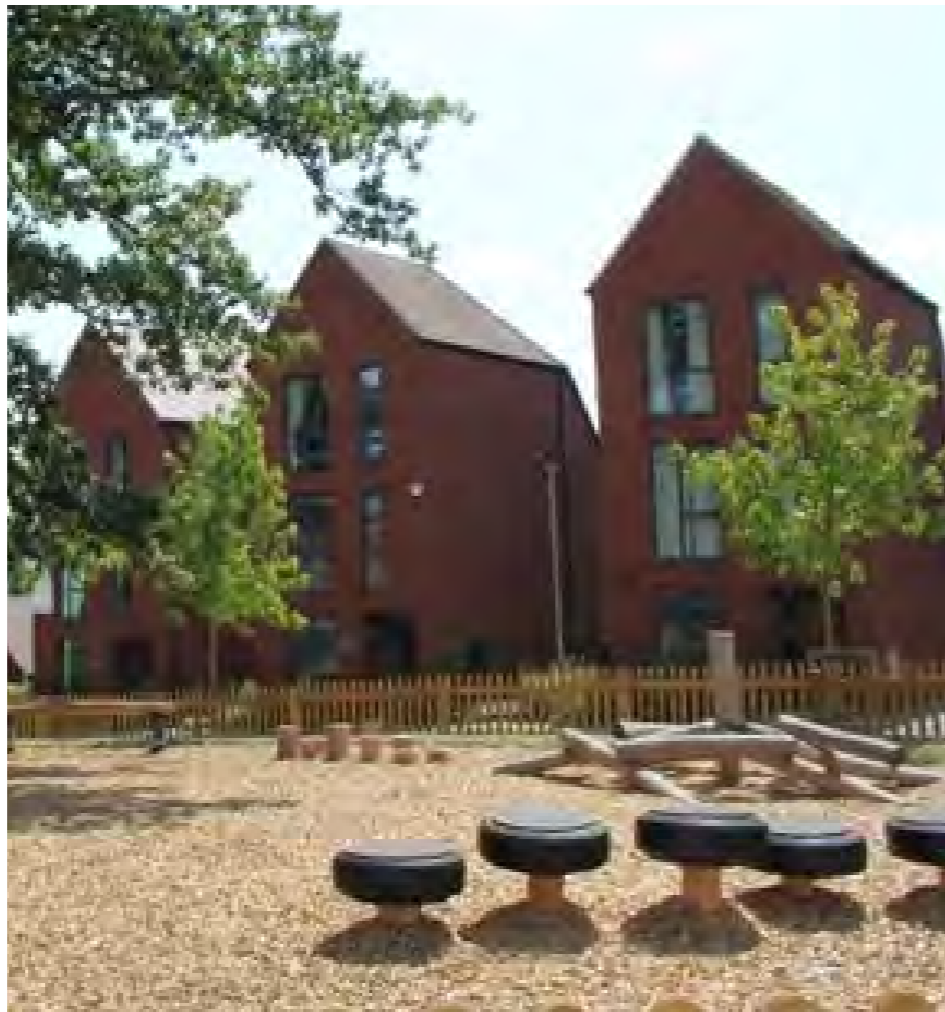
Figure 2.2a - Family homes with directly accessible amenity and play spaces
