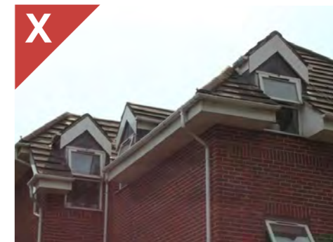
Figure 2.4.11f: Poorly proportioned and positioned of dormers and eaves results in a poorly resolved roof.
