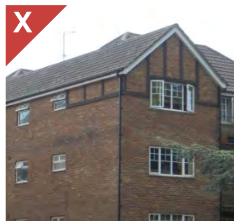
Figure 2.5.2j - 2.5.2k: Detailing that shows that the materials lack depth and are surface applied, resulting in unappealing appearances. On the left, the change in render colour at the corner contributes to a flimsy appearance. On the right, the half-timbering has been wrapped around the side of the building but stops at the first window. It should have either been continued along the length of the side of the building or kept to a higher level within the gable so it did not break the eaves line.
