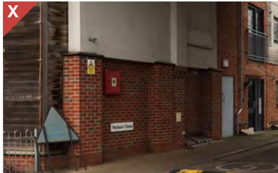
Figure 2.5.6a & 2.5.6b: Poorly considered placement of visible ancillary items on external envelopes
