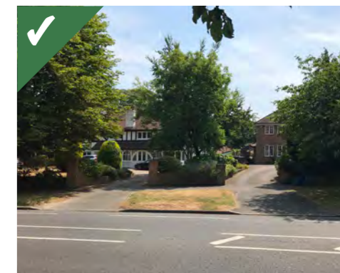
Figure 2.6.1c: Successful subdivision to provide a new home (right). The design of the entrance and boundary treatment, including planting, helps to integrate the newer dwelling into the streetscene.
