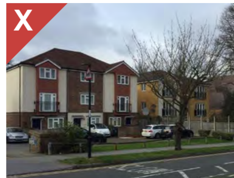
Figure 2.4.10d: A development which appears wide and squat as a result of poorly considered proportions and fenestration
