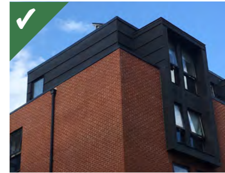
Figure 2.4.11a: Flat roof forms are acceptable. Set-back top floors with a change in material can be used to add interest and break down the mass.
