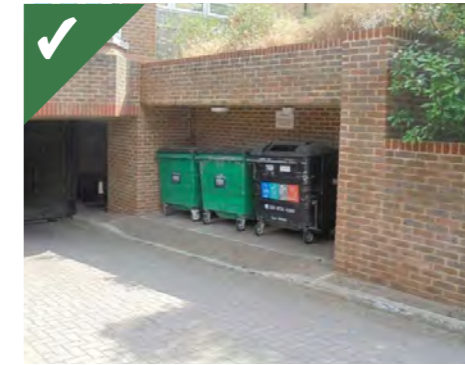
Figure 2.6.4d: A refuse store recessed within a boundary treatment conceals it from view from the street without the need for creating a separate structure. It could have been improved through the introduction of gates to enclose the front.
