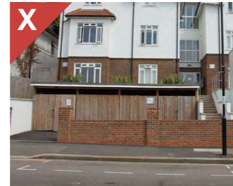
Figure 2.6.4b - 2.6.4c Refuse stores in highly visible locations that are not integrated into the landscape design or any other aspect of the design. The top image illustrates insufficient storage being planned for, resulting in bins cluttering the driveway.
