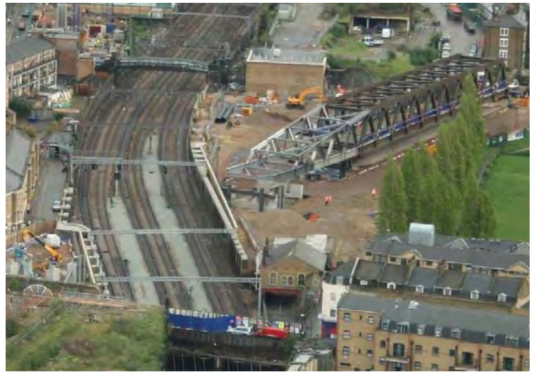
Push Launch construction technique used at GE19 bridge in Shoreditch, London
