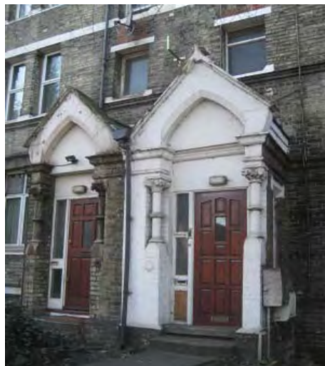
Projecting porches at Bellfield
