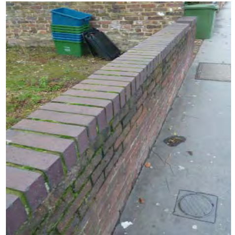
Modern brick low walling
