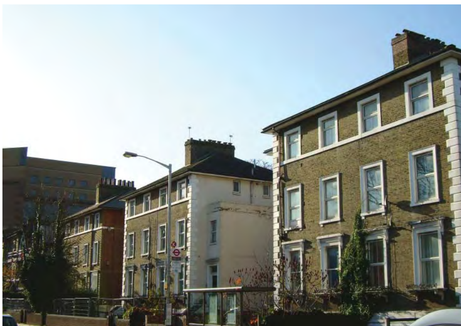
Buildings on the west side of Wellesley Road
