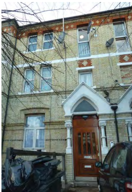
Newly cleaned facade of Belfield terrace
