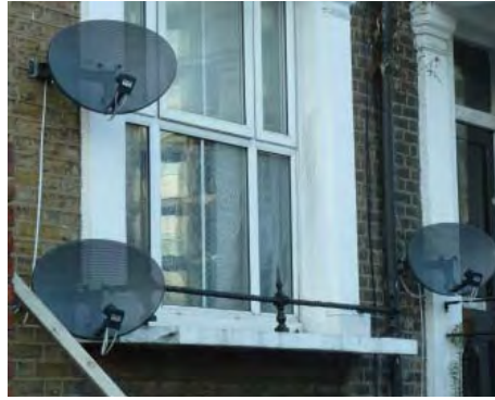
Multiple satellite dishes installed to the front elevation of a building
