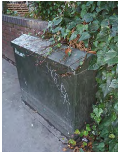
Telecommunications cabinet on the west side of Wellesley Road, adding to clutter on the pavements
