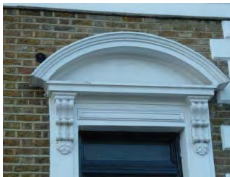
Segmentally pedimented doorway
