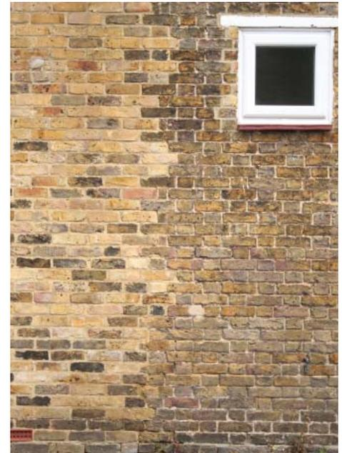
Photograph illustrating a poor matching of bricks for an extension with that of an existing building
