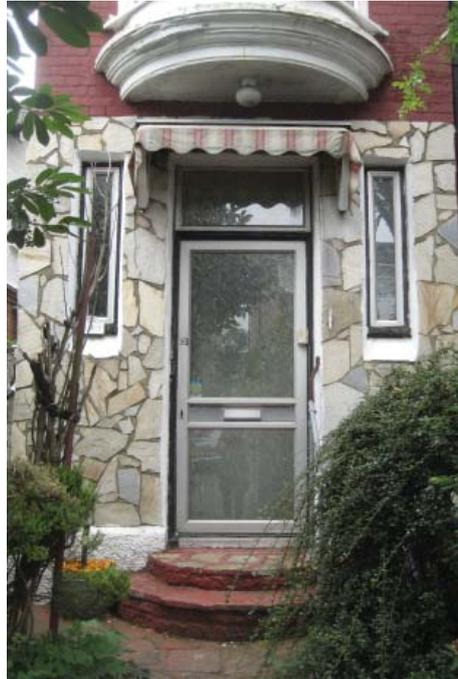
An example of inappropriate installation of an aluminium door. This development has harmed the character and appearance of the conservation area
