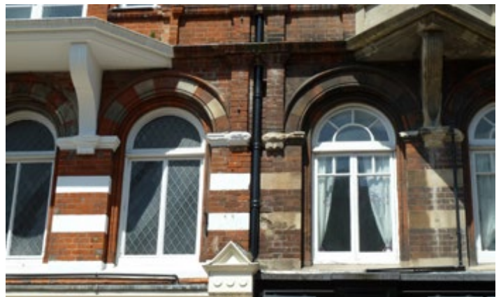
Cleaning and repainting (above left) can have a significant positive impact on a building's appearance
