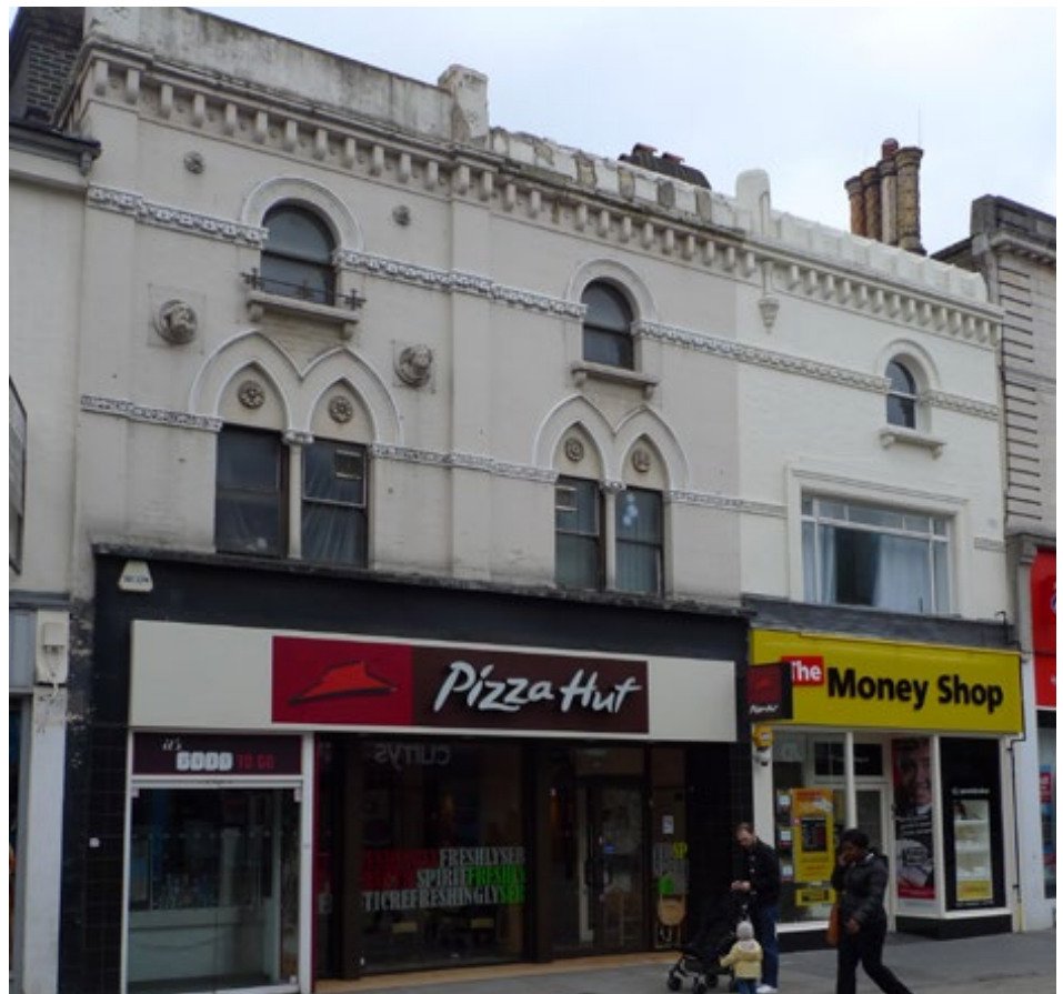
57-61 North End, locally listed. Unsympathetic window replacement and alteration to the window opening (above right) and a modern shop front and oversized fascia that disregards the character of the architecture above (above left)
