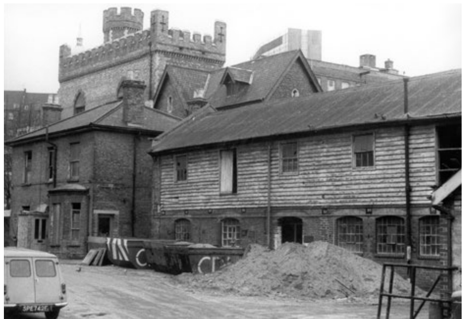
Historic photo c.1970s of the Surrey Street Pumping Station, which can be seen in the distance. The buildings in the foreground of this photograph have been demolished.
