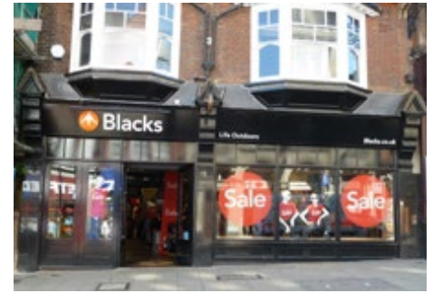
3-5 High Street: traditional style timber shopfront
