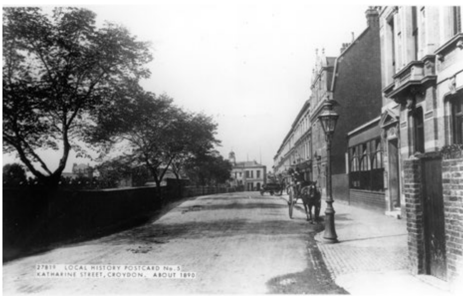
Katharine Street, 1890, looking towards the old Town Hall. The new Town Hall would be built on the left. The wall in the left foreground was above the former Central Station, now the sunken part of the Queens Gardens (see para 2.2.13)
