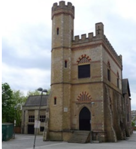
Surrey Street Pumping Station, Exchange Square, Grade II listed
