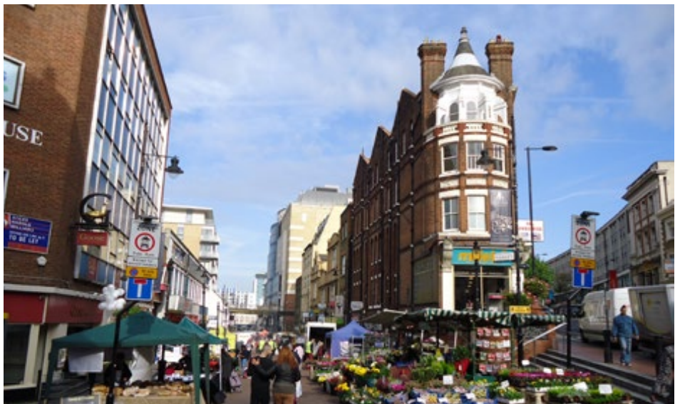
52-54 High Street (Millets building) at the sharp corner between Surrey Street and the High Street where there are significant land level changes
