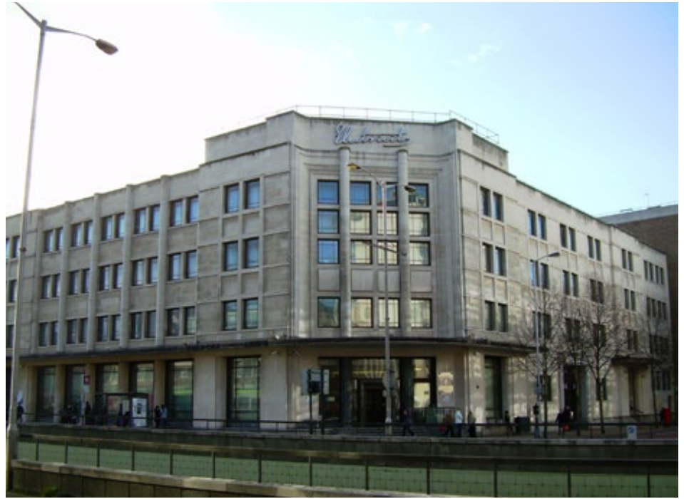
Electric House, Wellesley Road, Grade II
