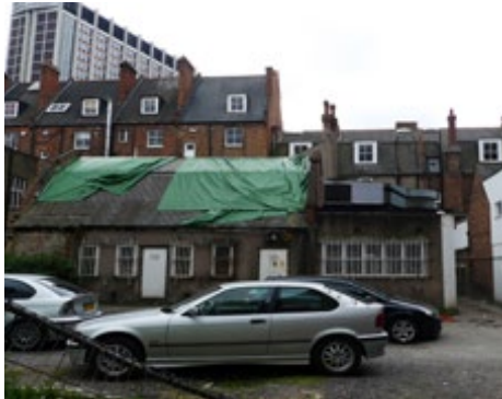
The rear of George Street is poorly maintained
