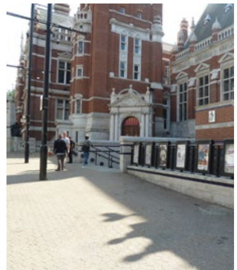
The Mid Croydon Masterplan includes a town square on Katharine Street opposite the Town Hall
