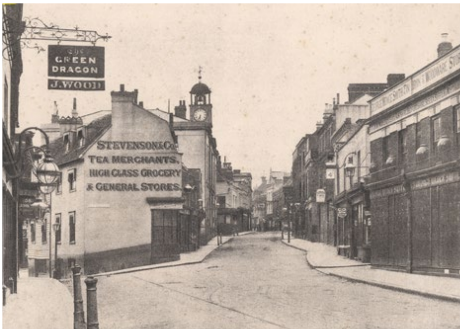
High Street 1890, before road widening (see Map 9 on p.16). Surrey Street is on the left and the clock tower is that of the old Town Hall on High Street. The Ship public house is on the right.
