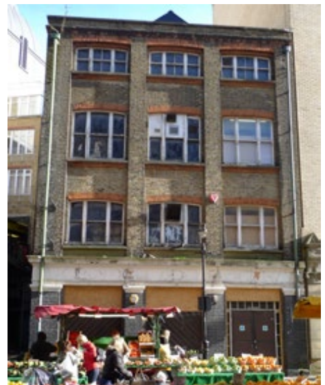
46 Surrey Street, the former Croydon Advertiser building, is currently in a poor condition
