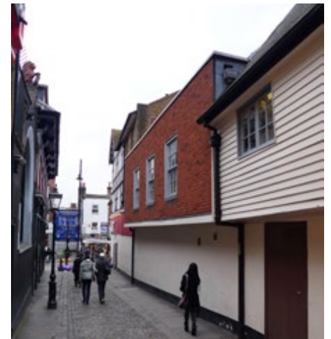
The rear of Numbers 11 and 13 Crown Hill, from Bell Hill
