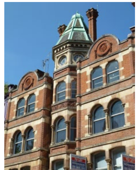
Detail of 32-34 High Street
