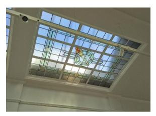
The original roof lights have been cleaned and repaired where necessary and allow natural light to flood in from the new glass roof above
