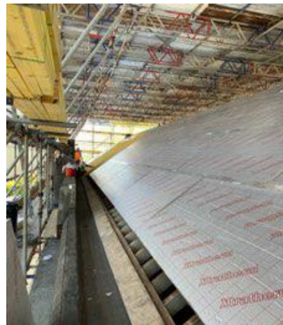
Roof insulation underway
