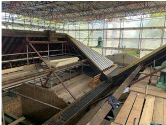
General view of progress to the roof
