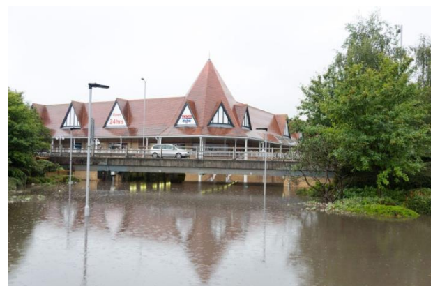
Figure 8 - 2015 Flooding at Purley Cross
