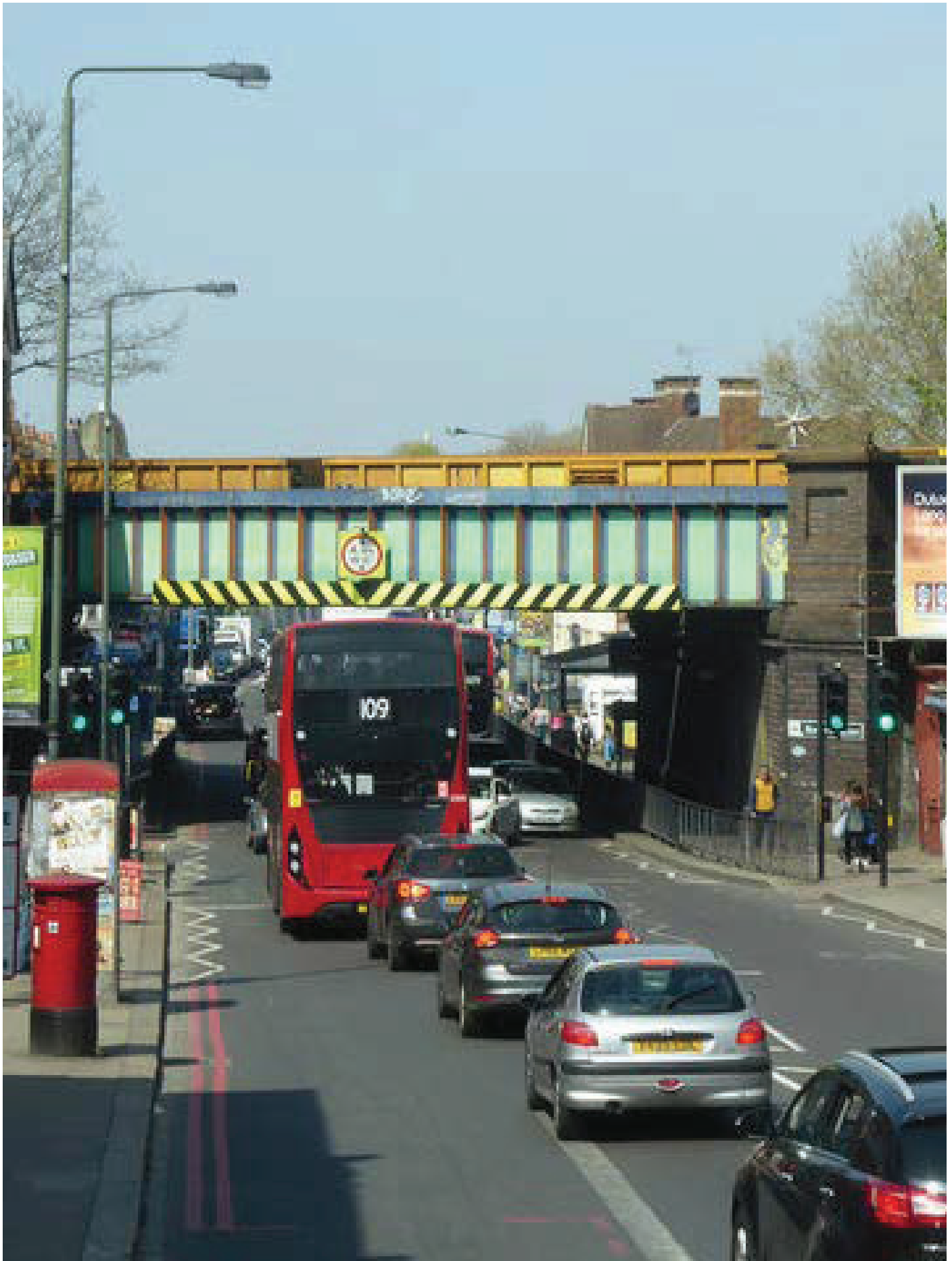
Existing View from South - Norbury Railway Bridge
