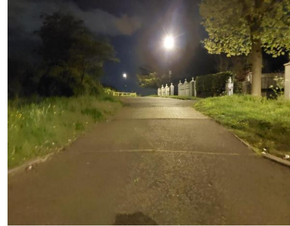
Photograph showing the street lighting dimming regime before and after implementation
