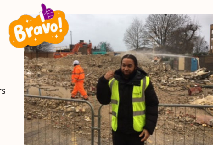
▲ Joshane on site at Regina Road
