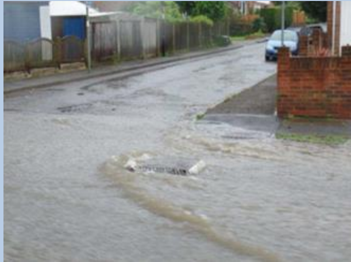
Figure 3 Surcharging manhole on Caterham Drive
