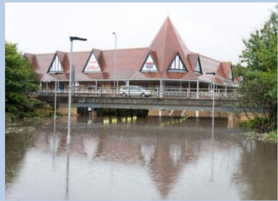
Figure 1 Purley Cross underpass (Croydon, 2015)
