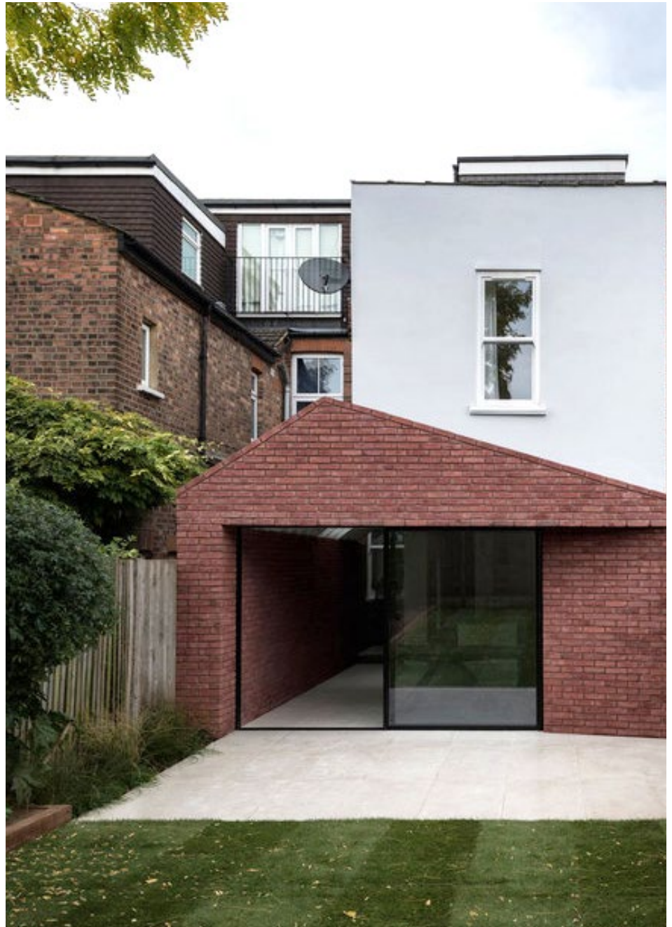
Figure 4.1b: An extension that successfully uses contemporary details and an un-symmetrical roof pitch to add interest to this design by Trehwela Williams. (Photo: Simone Bossi)
