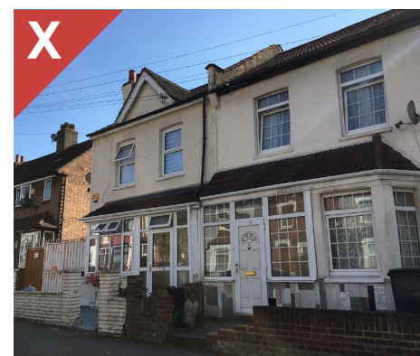
Figure 4.14b: A poor example of two porches that have been built up to and over original bay windows. The design fails to respond to the historic pattern of development and materials are low quality.
