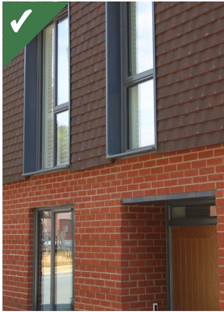
Figure 4.25a: A wall with different depths of window and door reveals. Deeper reveals add emphasis and solidity to the appearance of a house.
