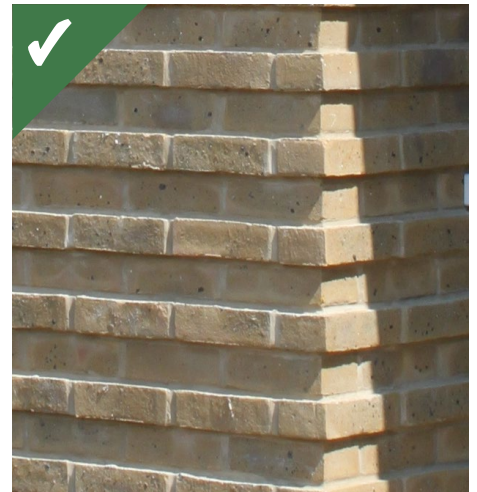
Figure 4.27e: Stepped courses of brickwork.
