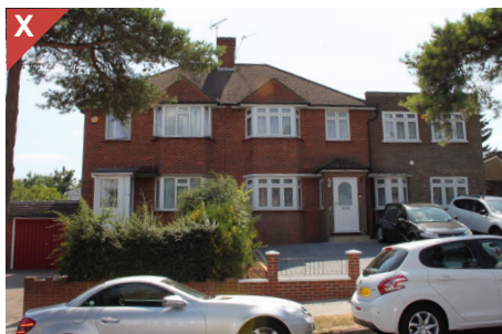
Figure 4.17b: A low quality two-storey side extension which is overly dominant, upsetting the balance of this pair of semi-detached homes. The brick neither matches nor distinguishes from the existing and the junction at the eaves is poorly detailed.
