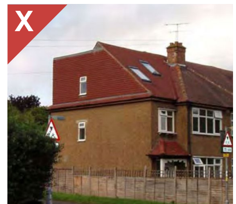
Figure 4.21g: Example of where a highly visible roof extension dominates the original building and negatively impacts the appearance of the street. This could have been avoided had the rear box extension been set in from the gable end of the roof to allow the gable and the rear extension to read as two separate elements.
