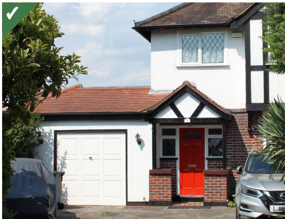
Figure 4.14a: Example of a good side extension wrapping around to incorporate a well-designed porch, successfully integrating with the existing dwelling.
