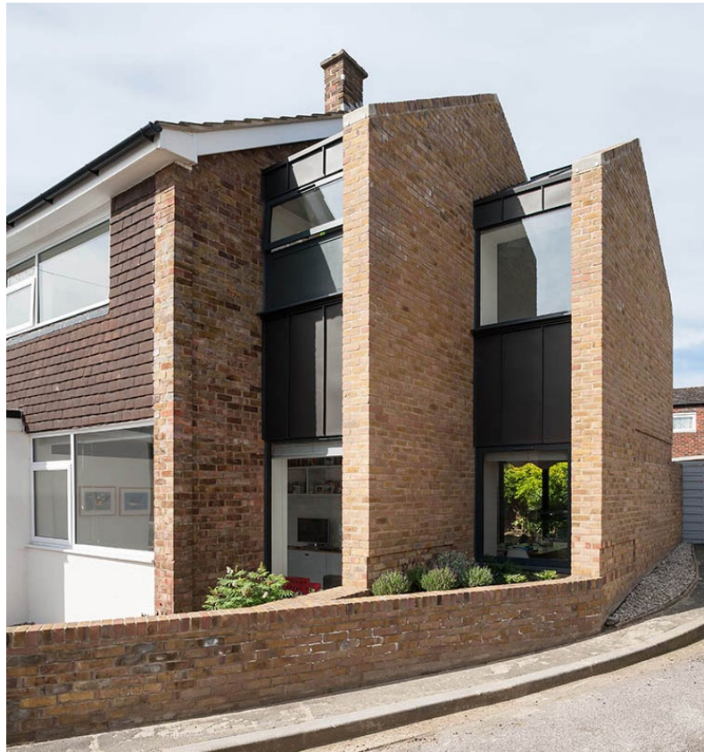
Figure 4.5a: A supplementary side extension designed by Selencky Parsons. The form clearly relates to the existing house, but successfully introduces larger windows and combines new materials with brickwork to complement the existing house. (Photo: Andy Matthews)
