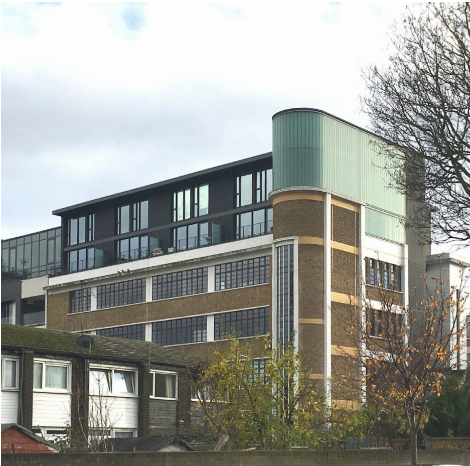
Figure 4.22a: An example of additional storeys being added to an existing building to provide new homes.
