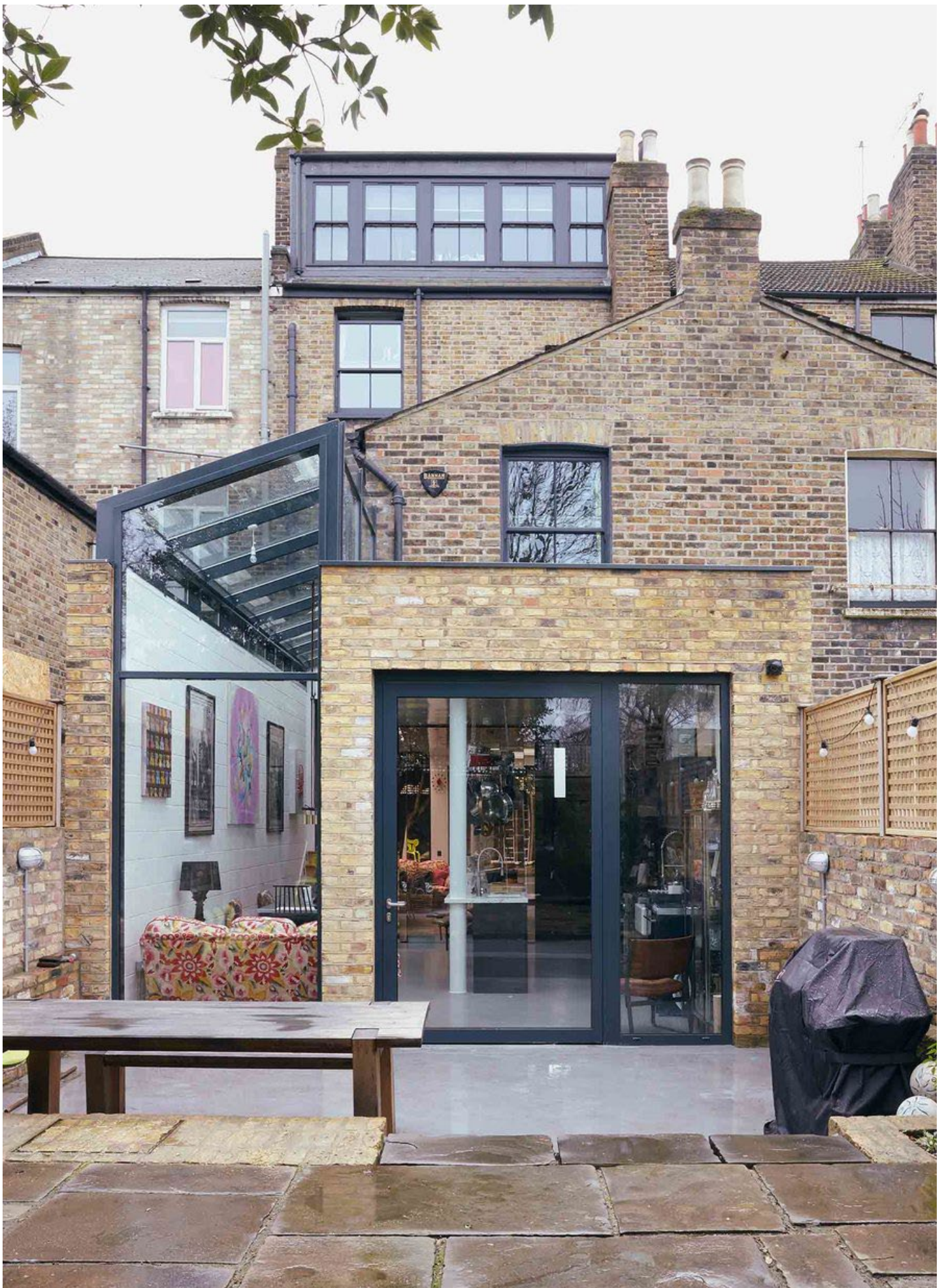
Figure 4.5c: A series of extensions designed by fourth_space that appear supplementary to the original house by clearly responding to its existing form and materials.
