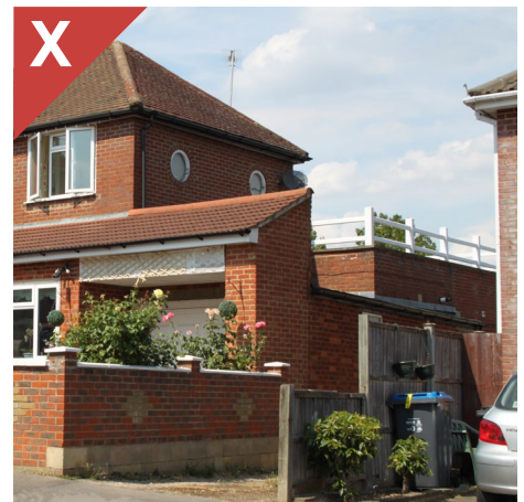
Figure 4.15b: A side and front extension with a series of different roof forms results in a poorly considered composition that has a negative impact on the streetscene.
