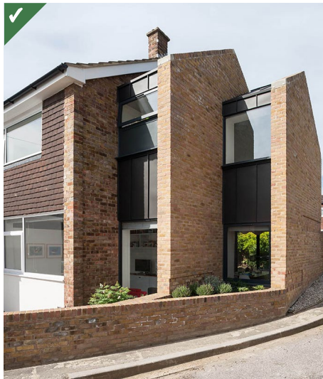
Figure 4.17c: Example of a subservient two-storey side extension designed by Selencky Parsons that introduces contemporary elements, such as the windows and their surrounds, to help distinguish the new from the existing. (Photo: Andy Matthews)
