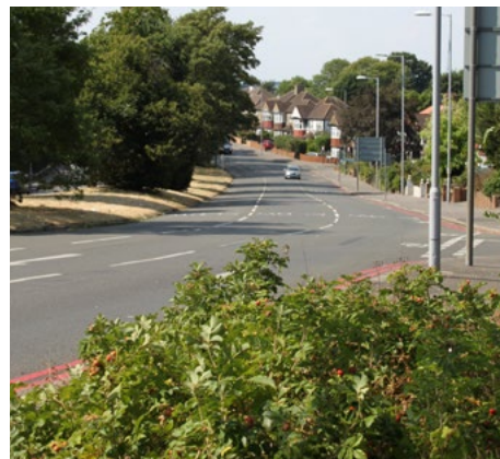
Figure 3.16b: A232 Dual Carriageway.
