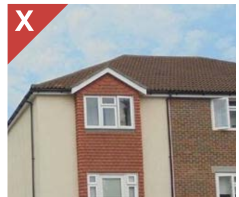
Figure 2.19f: Pitch of roof appears too shallow in relation to mass of building.
