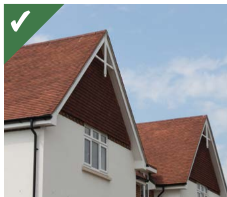
Figure 2.19e: Pitch of roof is steep enough to read positively in the streetscene.
