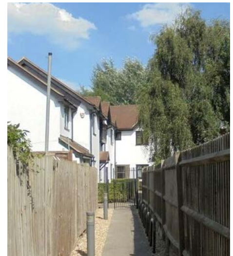
Figure 2.29h: A new route created by a back land development is well lit, overlooked and has a legible destination.
