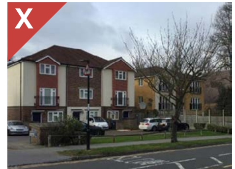
Figure 2.17d: A development which appears wide and squat as a result of poorly considered proportions and fenestration.
