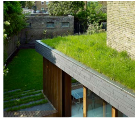
Figure 2.36a: Green roof designed by Hayhurst & Co.
