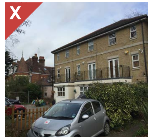
Figure 2.24b: Windows are too small and their positioning fails to break up mass of façade.
