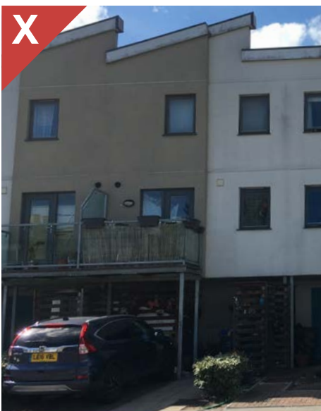
Figure 2.26a: External balconies with supports that are not integrated into design of the proposal. The use of glass balustrades have resulted in occupiers retrofitting screening devices to provide privacy that exacerbates the poor appearance.
