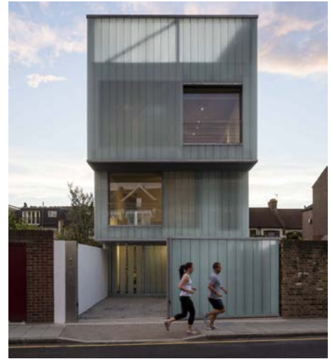
Figure 2.22a: An innovate material approach to an infill development by Carl Turner Architects. (Photo: Tim Crocker)
