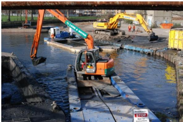
The Environment Agency funded a dredging programme which was completed in early 2009. The task to remove urban sediment and other matter from the canal over a distance of 3.2kms was completed over a 3 month period at a cost of £2million. As a result of the initiative over 30,000 m<sup>3</sup> of sediment was removed in addition to 3 tonnes of tyres, 3 cars, 40 motorbikes and 120 shopping trolleys.
