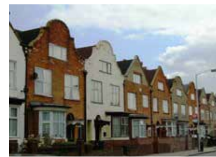
Photo 93. Terraced houses on Melfort Road
