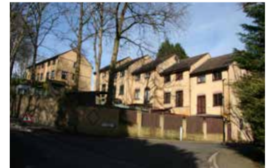
Photo 47. Compact houses on relatively small plots along Sylvan Hill
