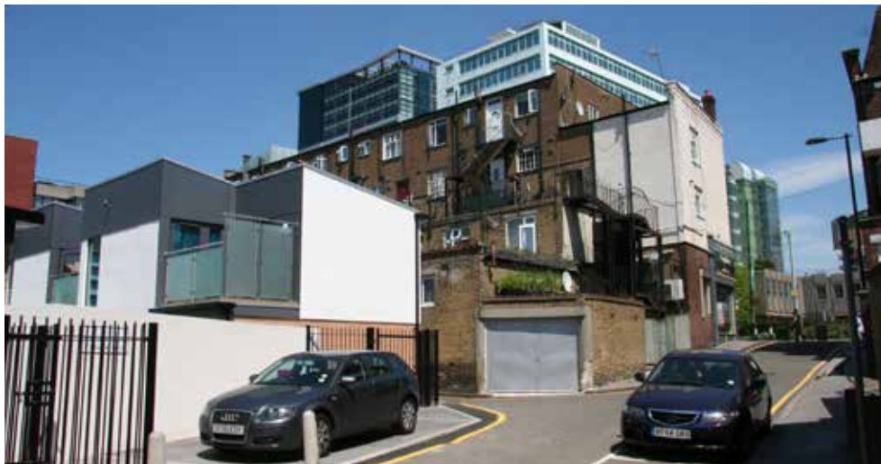
Photo 41. New in-fill residential development at Meadow Stile
