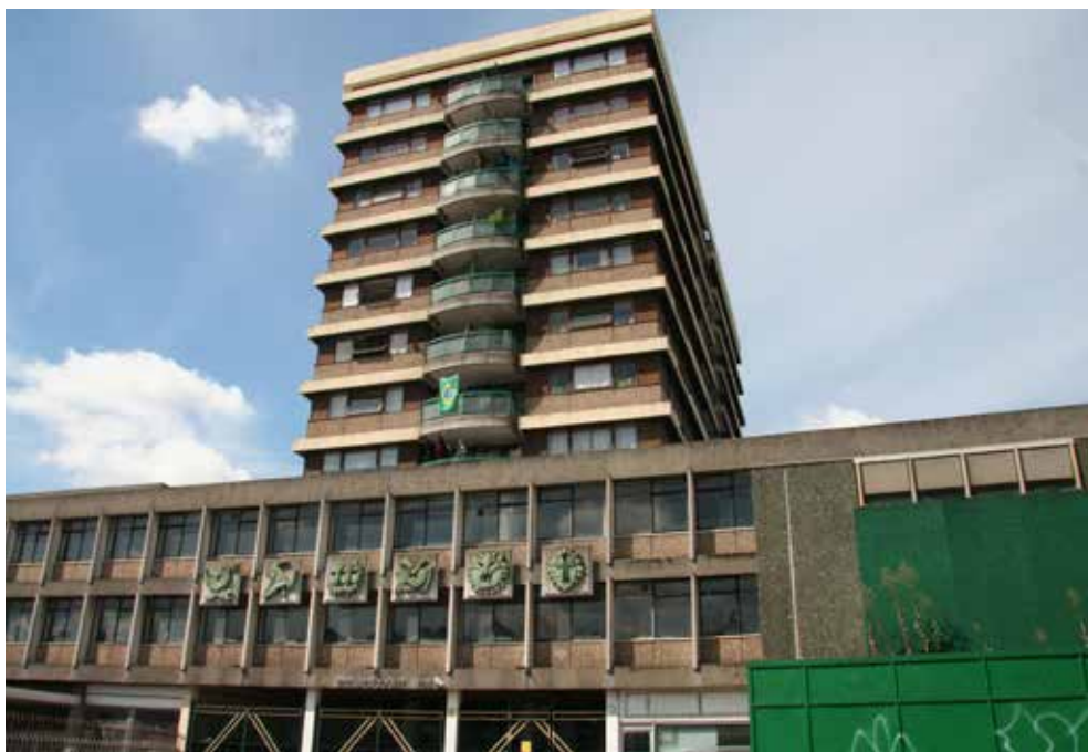
Photo 9. Large buildings on London Road: Zodiac House
