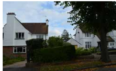
Photo 59. Box Ridge Avenue
