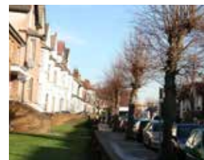
Photo 14. Larger residential terraces
