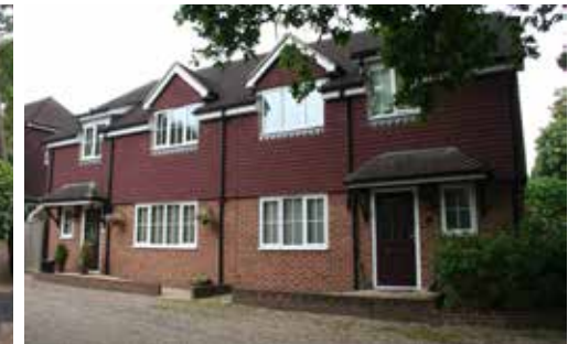
Photo 76. Compact houses on Upper Shirley Road
