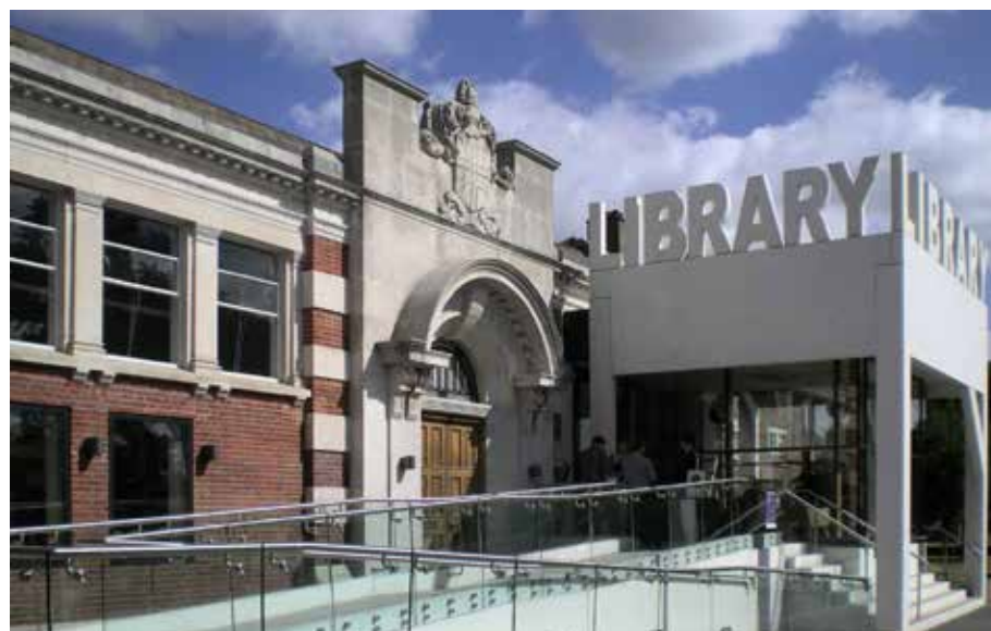
Photo 91. Thornton Heath Library
