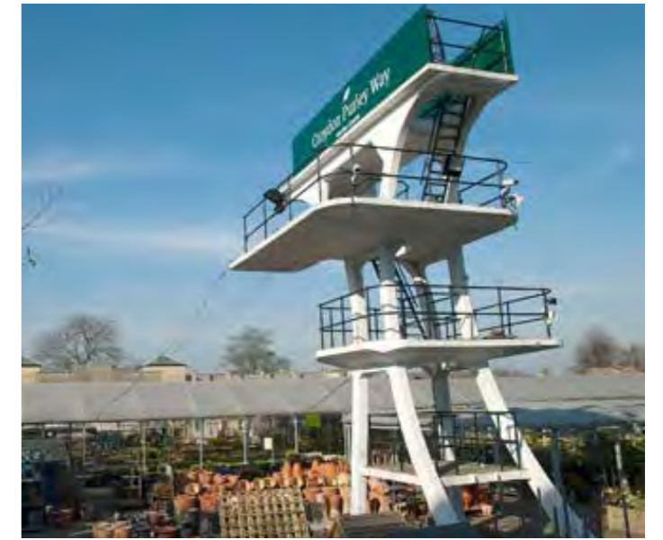
Listed diving board from former Lido, now in Garden Centre site
