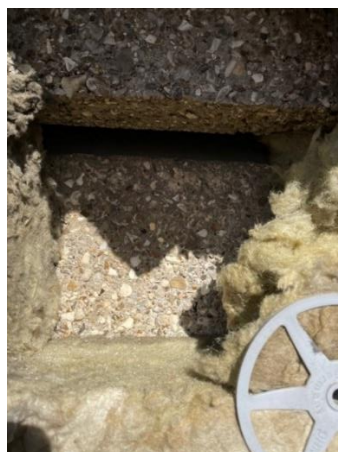
Figure 12. Location 1.1 gap identified behind existing infill panel
