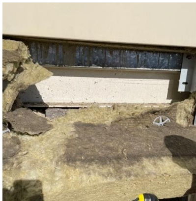
Figure 36. Location 3.1 steel beam behind mineral wool insulation
