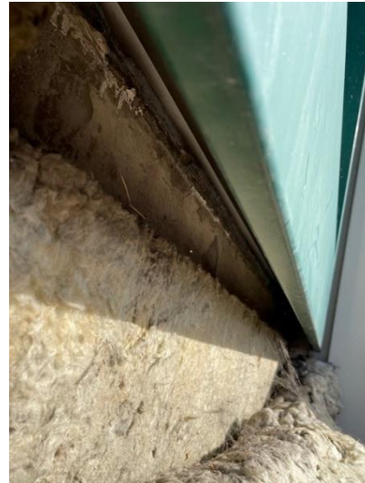
Figure 15. Location 1.3 existing window frame behind aluminium cladding
