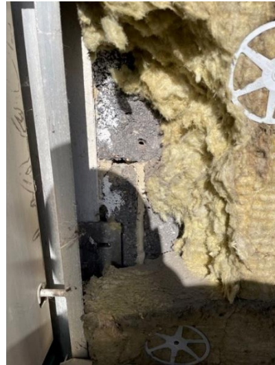
Figure 35. Location 3.1 100mm insulation with blockwork behind
