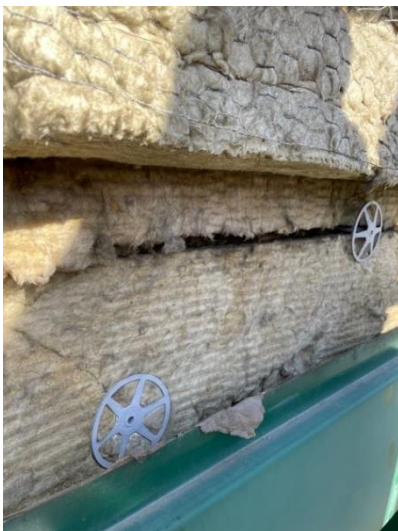
Figure 20. Location 1.5 horizontal cavity barrier
