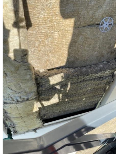
Figure 26. Location 1.7 horizontal cavity barrier at floor level
