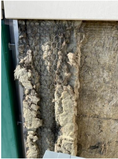
Figure 30. Location 2.1 damaged vertical cavity barrier unlikely to be under compression
