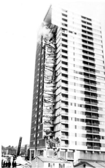
Figure 4. Ronan point collapse
