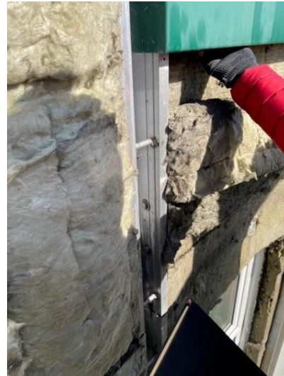
Figure 19. Location 1.4 horizontal cavity barrier under window
