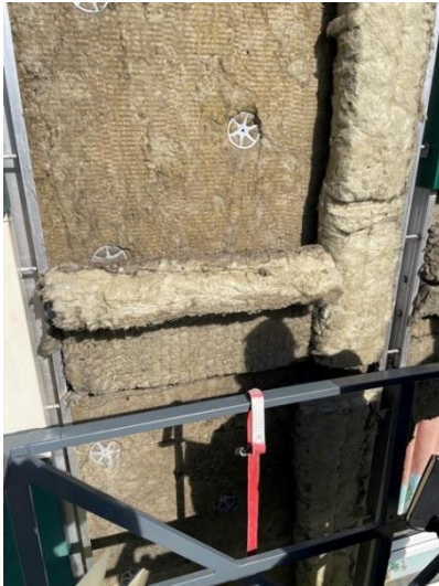
Figure 18. Location 1.4 horizontal cavity barrier at floor level – not folded over completely
