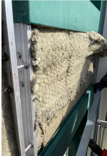
Figure 14. Location 1.3 horizontal cavity barrier under flat window
