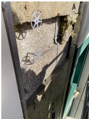
Figure 10. Location 1.1 no horizontal or vertical cavity barrier
