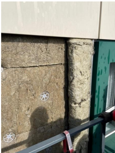
Figure 16. Location 1.4 vertical cavity barrier in place
