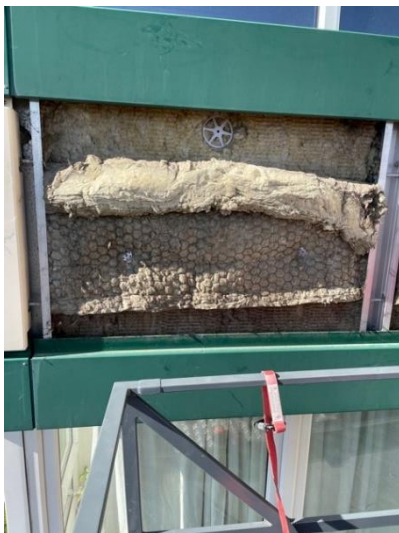
Figure 32. Location 2.2 horizontal cavity barrier
