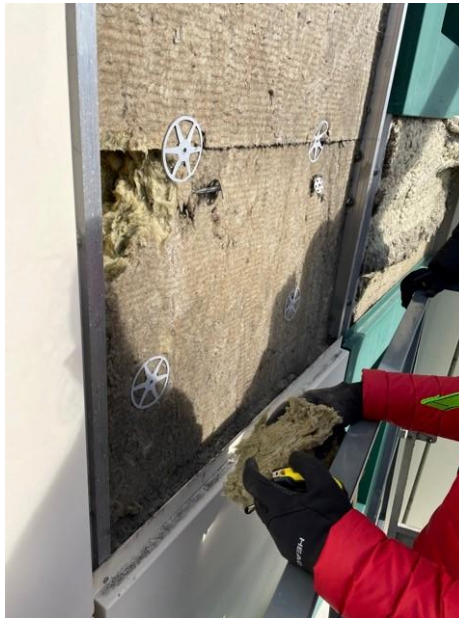
Figure 13. Location 1.2 there was no horizontal cavity barrier identified at floor level.
