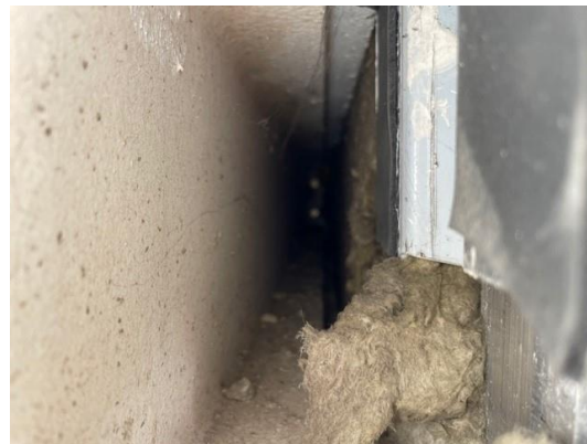
Figure 37. Location 3.1 steel beam (left) with insulation and panel (right) and unbroken cavity
