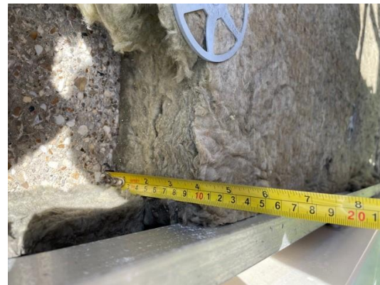
Figure 11. Location 1.1 100mm mineral wool insulation
