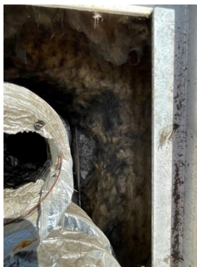
Figure 23. Location 1.6 cavity barrier enclosing ductwork (reinforced mineral wool)
