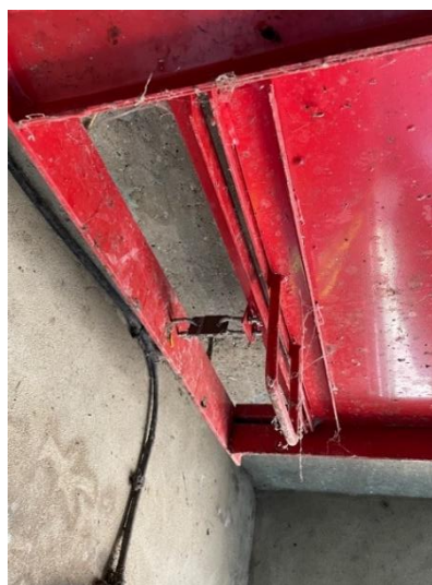
Figure 41. Bin chute fusible link
