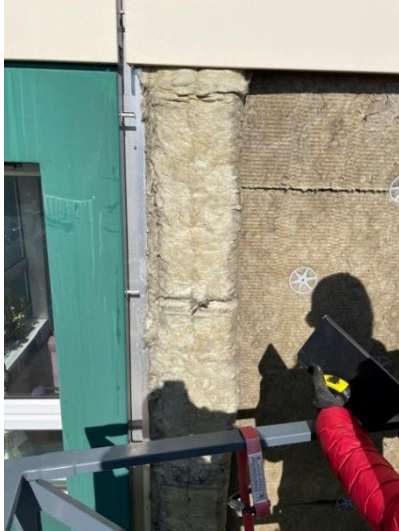
Figure 25. Location 1.7 vertical cavity barrier between window and continuous strip of cladding
