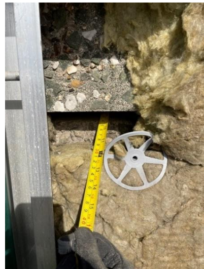
Figure 17. Location 1.4 gap identified behind concrete infill panel
