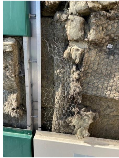
Figure 31. Location 2.1 damaged vertical cavity barrier not full fill and unlikely to be under compression
