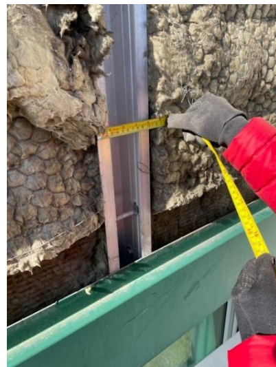
Figure 33. Location 2.2 100mm gap between cavity barriers
