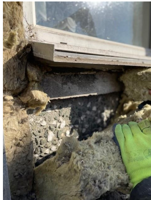
Figure 15. Location 1.3 original window frame behind insulation. A drip tray from the window can be seen.
