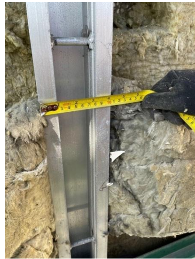
Figure 27. Location 2.2 100mm gap between cavity barriers
