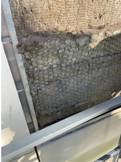
Figure 12. Location 1.2 non continuous cavity barrier at floor level
