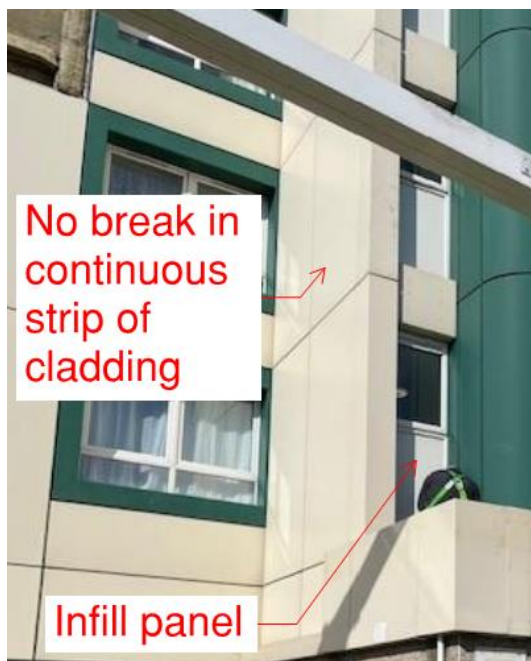
Figure 32. Location 4 – no horizontal barriers were found in this section of the cladding.
