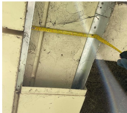
Figure 30. Location 3 300mm concrete beam
