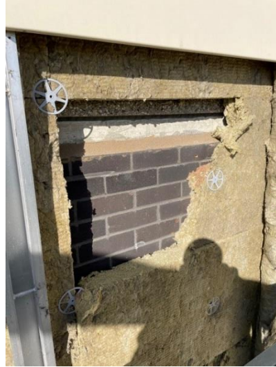
Figure 24. Location 2.1 masonry construction behind mineral wool insulation
