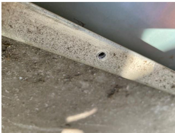
Figure 31. Location 3 solid aluminium panel 3-5mm thick
