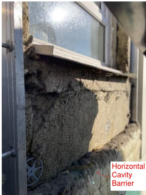
Figure 14. Location 1.3 horizontal cavity barrier
