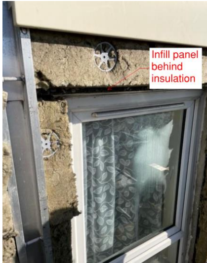
Figure 16. Location 1.3 no cavity barrier above window
