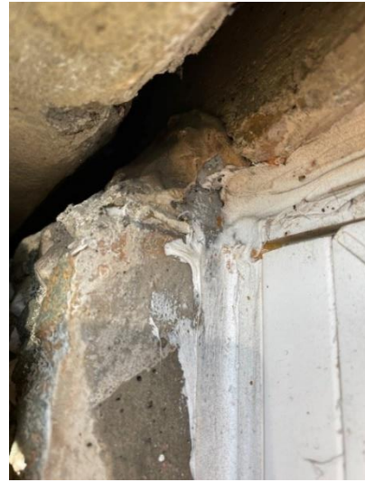
Figure 17. Location 1.3 gap between infill panel and structure behind
