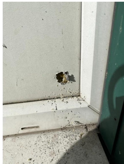
Figure 33. Location 4 hole drilled. It appeared to be a thermo plastic infill between two layers of steel.
