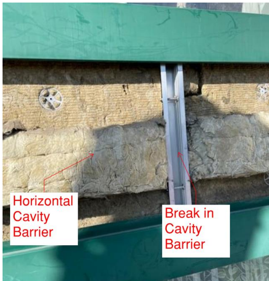
Figure 26. Location 2.2 cavity barrier under window
