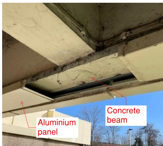
Figure 29. Location 3 structural beam enclosed in aluminium panel
