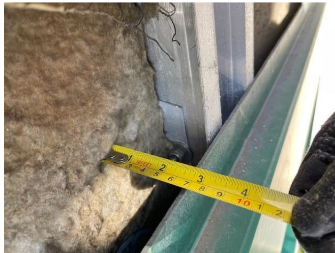
Figure 28. Location 2.2 60mm cavity
