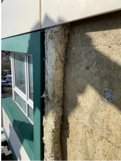
Figure 23. Location 2.1 vertical cavity barrier between window and continuous strip of cladding
