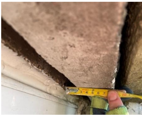
Figure 18. Location 1.3 30mm gap behind infill panel
