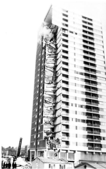
Figure 4. Ronan point collapse
