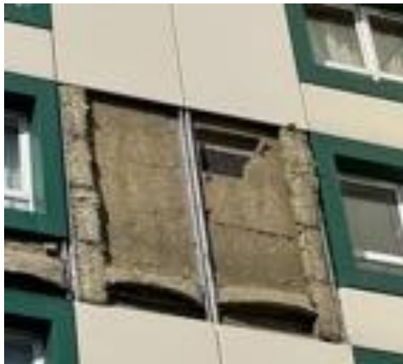
Figure 25. Location 2.1 vertical cavity barriers on either side of the continuous strip of cladding between windows
