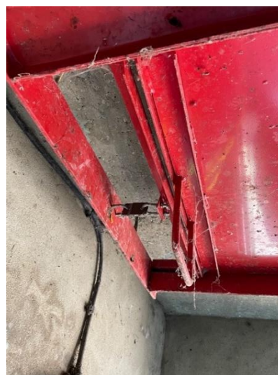
Figure 35. Bin chute fusible link
