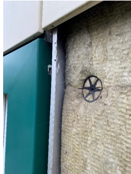
Figure 19. Location 2.2 vertical cavity barrier around the window
