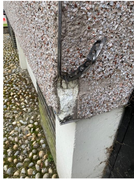
Figure 24. Location 3 exposed EPS behind stone render approximately 60mm deep to concrete.
