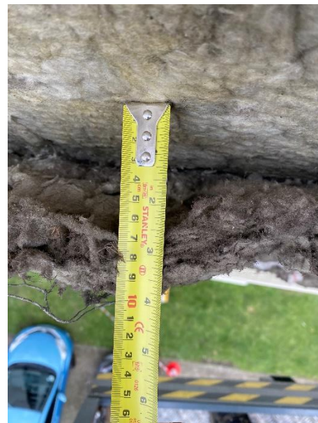
Figure 11. Location 1.1 cavity between insulation and cladding rails
