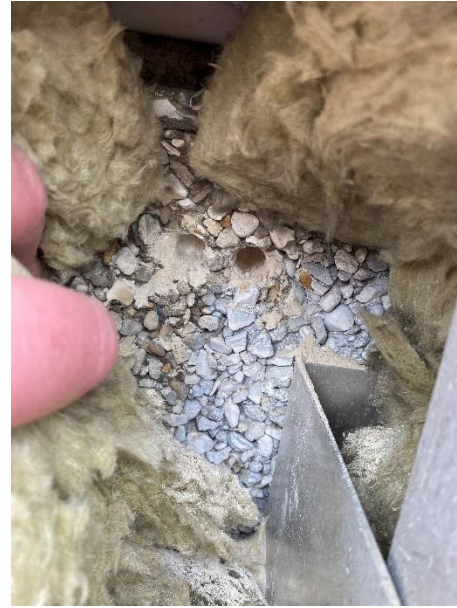
Figure 22. Location 2.3 approximately 25mm drill holes to concrete
