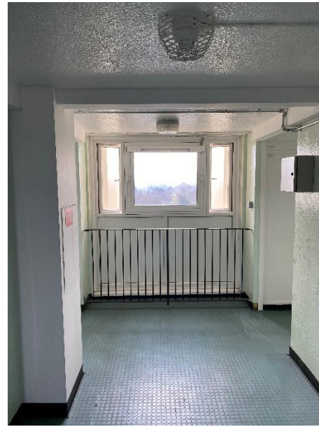
Figure 26. Location 4 lobby windows and infill panels below AOV
