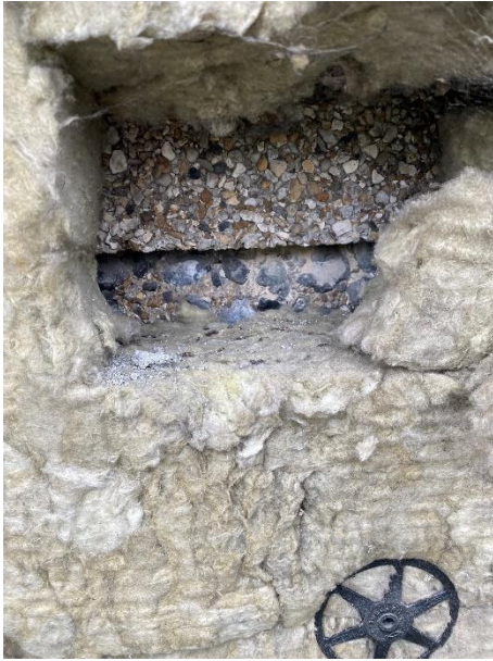
Figure 14. Location 1.3 original RC LPS construction behind overcladding and insulation
