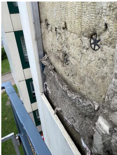
Figure 10. Location 1.1 no vertical cavity barrier
