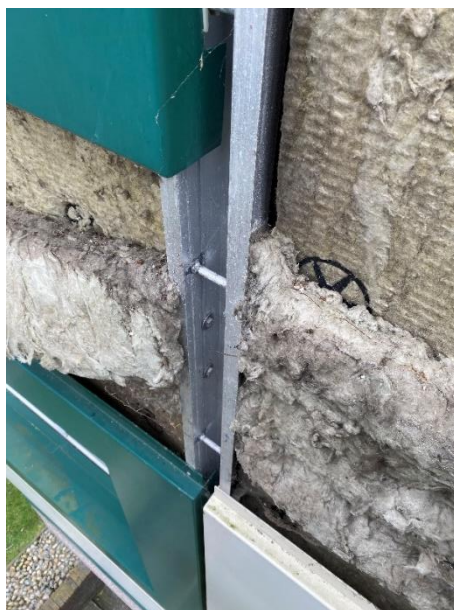
Figure 17. Location 2.1 horizontal cavity barrier around the corner
