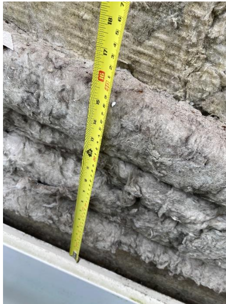
Figure 20. Location 2.2 horizontal cavity barrier at approximately slab level. The cavity barrier has not been folded and was not installed under compression.
