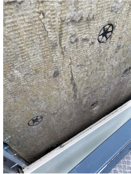
Figure 15. Location 1.3 no horizontal cavity barrier at slab level
