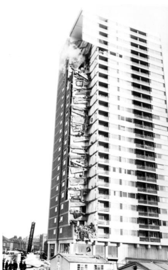
Figure 3. Ronan point collapse
