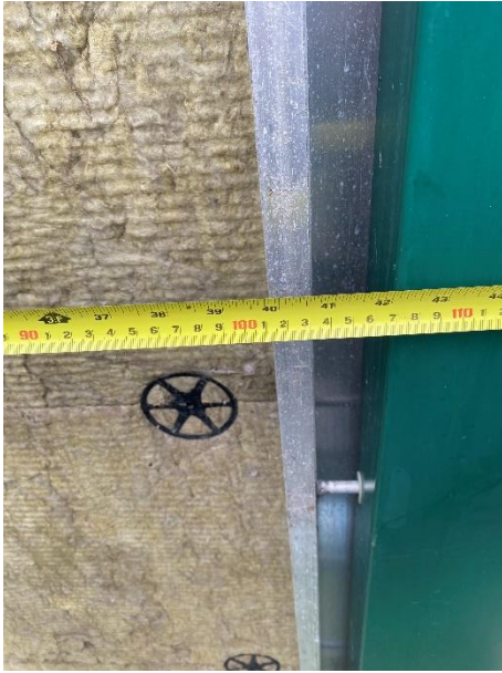
Figure 21. Location 2.3 no vertical cavity barrier around window
