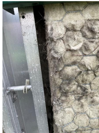
Figure 16. Gaps around cavity barrier at carrier system
