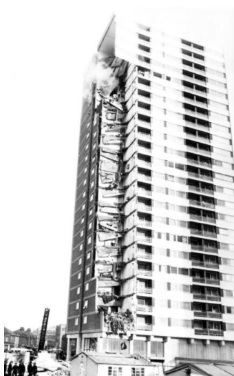
Figure 5. Ronan point collapse
