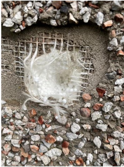
Figure 12. View of cladding and render system
