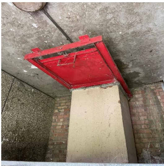
Figure 28. Bin chute damper with fusible link in bin store
