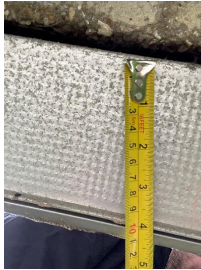
Figure 13. measurement of cladding where lintel was provided at base
