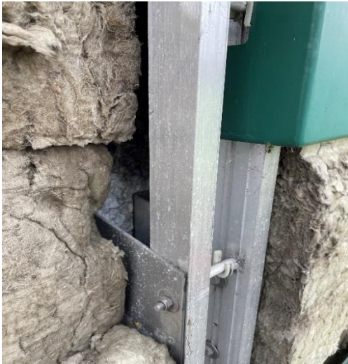
Figure 21. Gap in rockwool at carrier system
