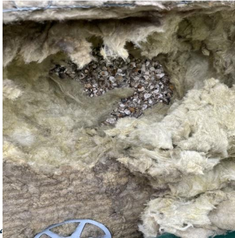
Figure 25. Render behind rockwool
