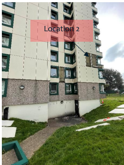
Figure 15. Metal cladding at 3 rd floor corner
