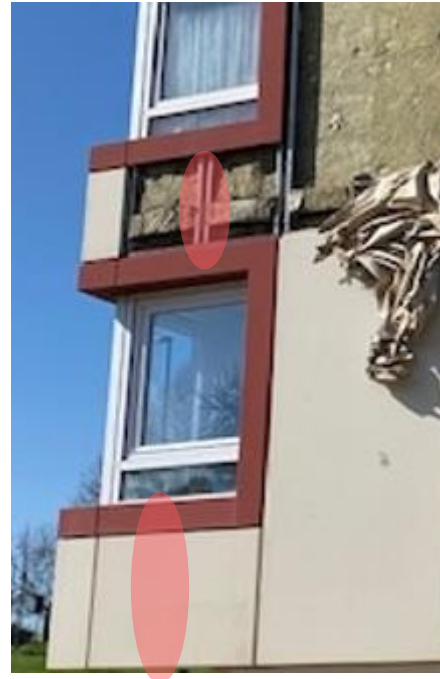
Figure 13. Location 1.1 – the highlighted areas show where the panel is fixed over the rail.
