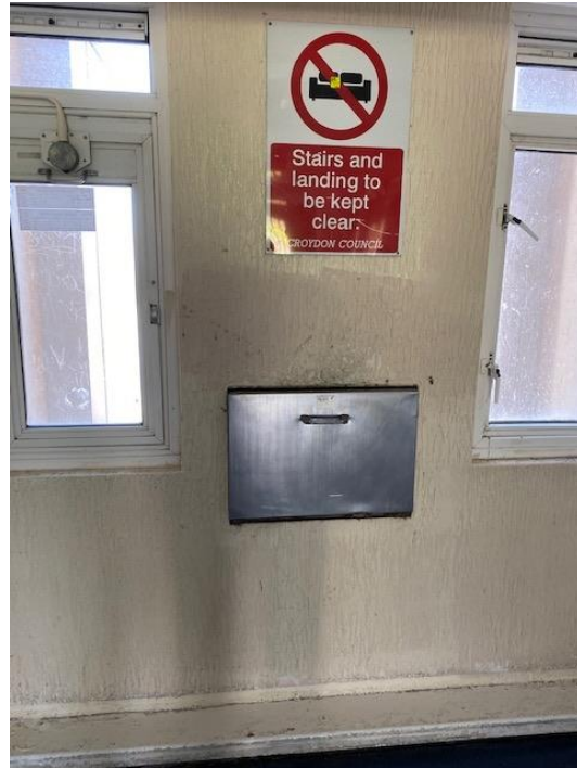
Figure 32. Typical bin chute hopper. An AOV can be seen to the top left.
