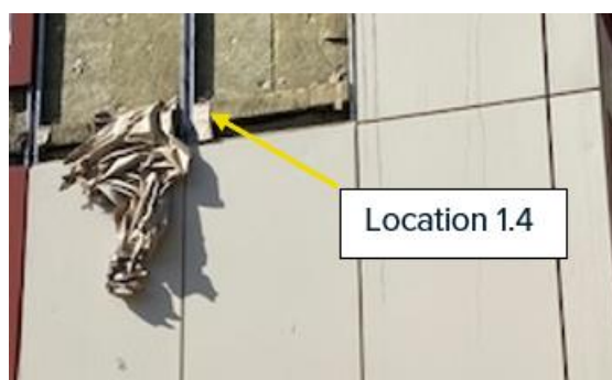
Figure 18. Location 1.4 – Cavity barriers are in place but are not under compression
