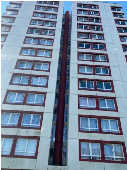
Figure 33. Showing the rubbish chute on the north face of the building
