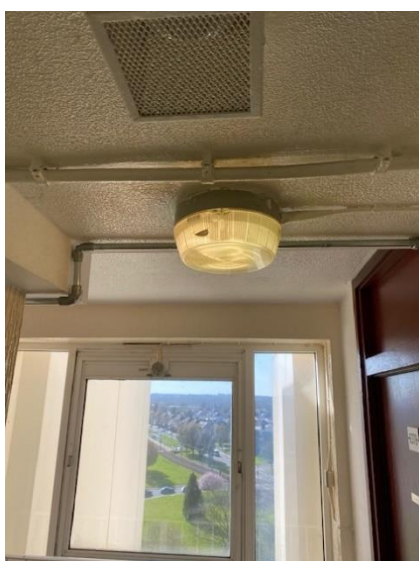
Figure 27. AFD (in wire cage) which operates the AOV in the lobby
