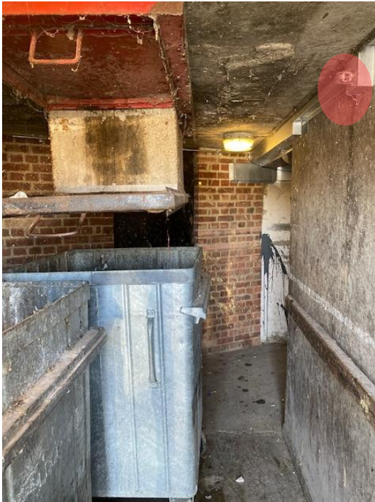
Figure 31. Showing sprinkler head (highlighted) and the spring loaded fire shutter over the wheelie bin
