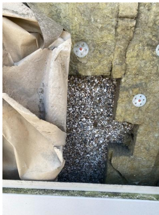
Figure 23. Location 2.2 showing the upper extent of the missing insulation
