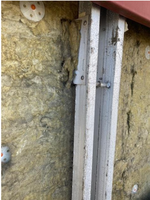
Figure 12. Location 1.1 - Location 1.1 - 100mm break in cavity barrier for an aluminium bracket
