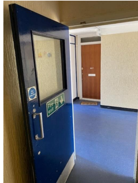
Figure 36. Lobby door on the ninth floor with a missing self closer.
