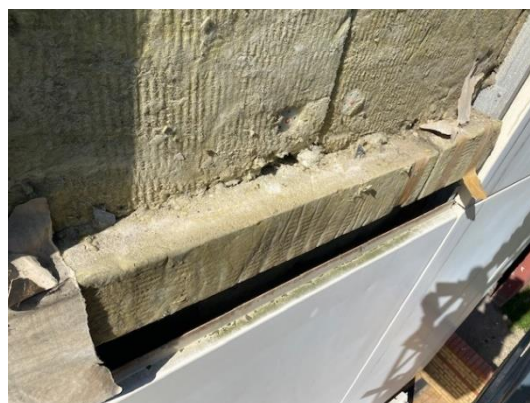
Figure 19. Location 1.4 – Close up of what appears to be a cut off section of material rather than an intended barrier product.
