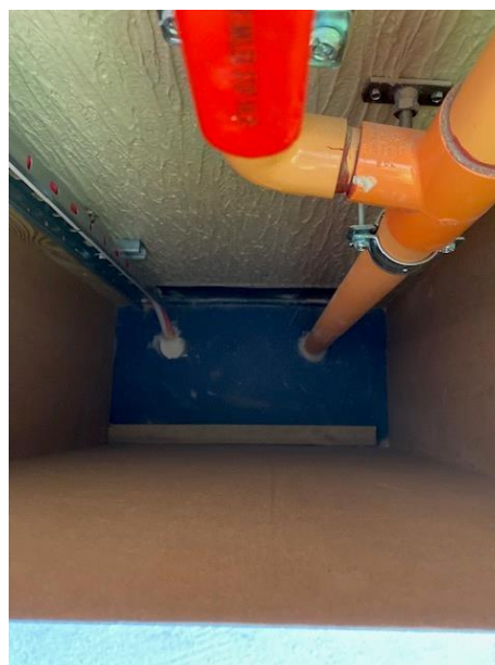
Figure 30. showing where the sprinkler pipe passes through the compartment floor.
