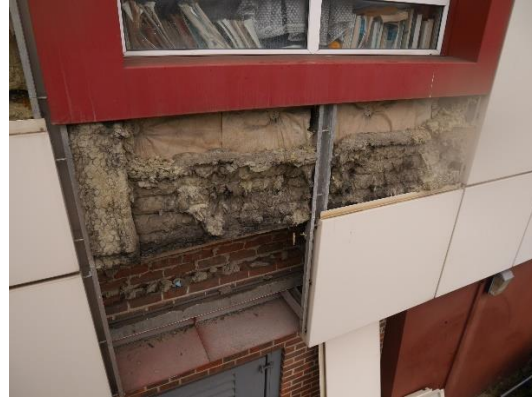
Figure 29. Location 1.7 Cavity barriers at this location are positioned above floor slab level against the cladding. They do not form compression against the cladding panels. The soffit is a 2mm metal panel.
