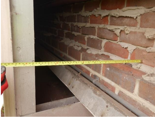
Figure 28. Location 1.7 The soffit provides what appears to be an undivided gap around the building of 470 - 500mm wide x 750mm high.
