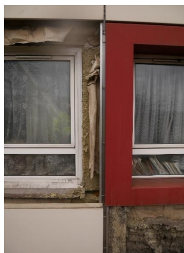
Figure 23. Location 1.5 A vertical compartment barrier is shown at the right-hand side of the party wall location. There is evidence of water damage to the insulation on the left-hand side. Cavity barriers around windows have not been installed but were not required by building regulations at the time of the over cladding works.
