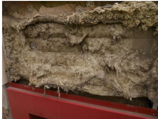
Figure 31. Location 2.1 Horizontal cavity barrier at second floor level which does not provide compression against the cladding panel face. Evidence of vermin route across the top of the barrier.
