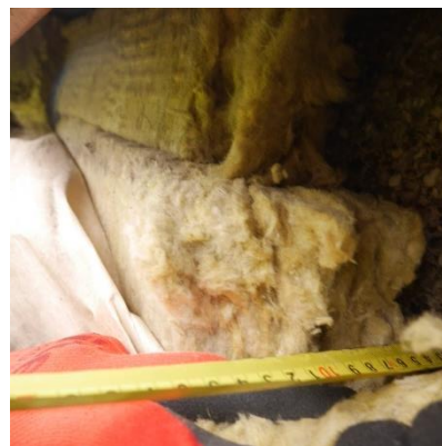
Figure 11. Location 1.1 100mm mineral wool insulation.
