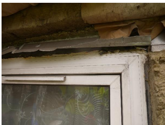
Figure 20. Location 1.5 The original head flashing has been peeled back to allow window replacement.
