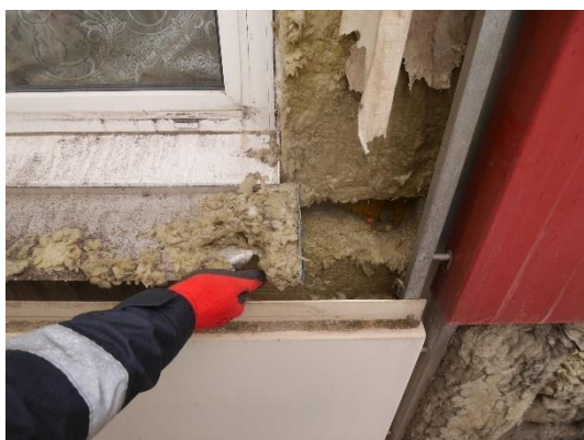
Figure 20. Location 1.5 The original head flashing has been peeled back to allow window replacement.
