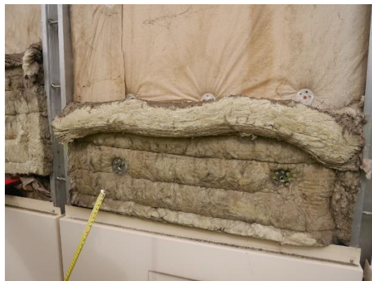
Figure 14. Location 1.2 line of horizontal cavity barrier at floor level, barrier is not folded over and only in partial compression at the head.
