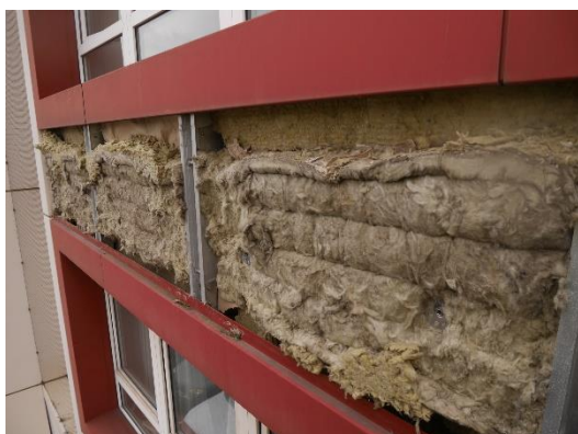
Figure 34. Location 2.3 Horizontal cavity barrier at first floor level, there is little or no compression against the cladding panels.
