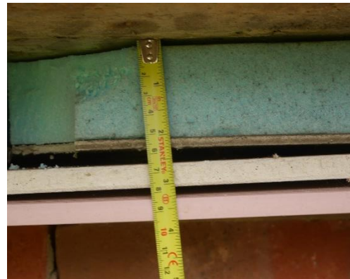
Figure 27. Location 1.7 The first-floor slab has been underdrawn with a cement particle board backed with foam insulation, further underclad with two layers of what appear to be pink plasterboard.
