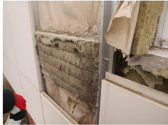
Figure 25. Location 1.6 cavity barrier at side of window (horizontal barrier), this is located at a higher level above the slab level but against concrete panels. It is not folded over and provides only minimal compression against the cladding at the head.
