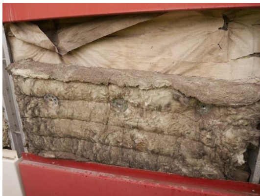
Figure 10. Location 1.1 horizontal cavity barrier at floor level, barrier has not been folded over and is not in compression against the cladding.
