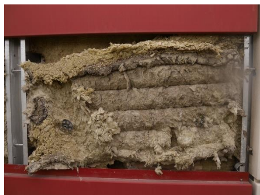
Figure 35. Location 2.3 Section of barrier shows vermin routes both horizontally and vertically against the cladding panel.
