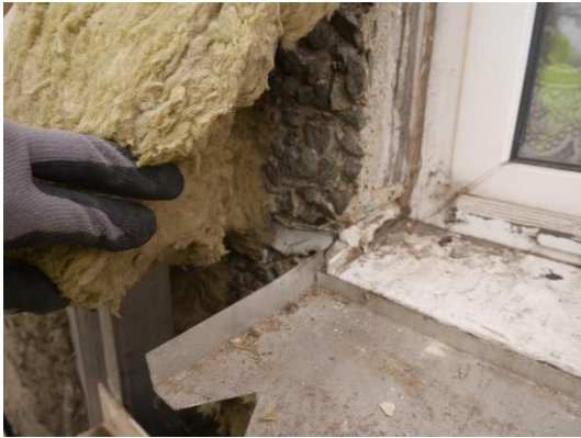
Figure 24. Location 1.6 Window jamb, shows original concrete panels with panel joint seal intact, mastic seal around window is from the time of replacement and not thought to be a fire seal.
