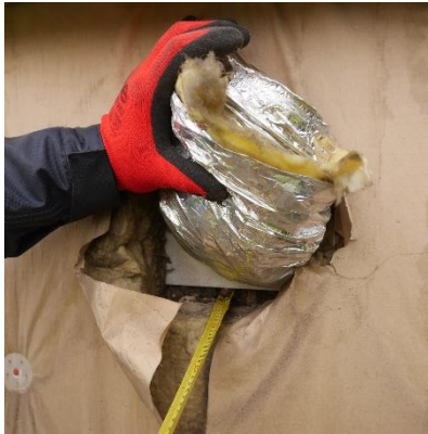
Figure 15. Location 1.3 ventilation duct and back plate surround. Building paper facing is visible over mineral fibre insulation.
