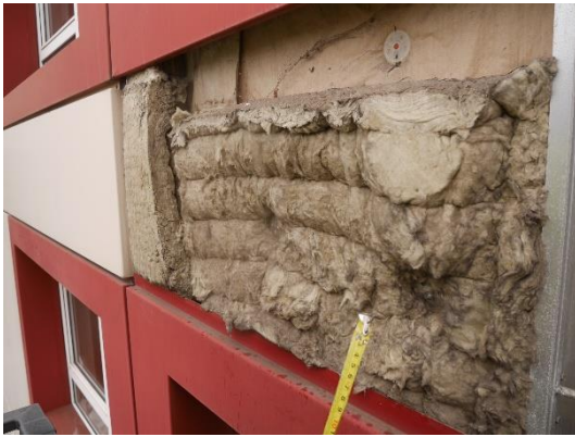
Figure 17. Location 1.4 Horizontal cavity barrier at floor level, a vertical compartment barrier is located on the left hand side of the panel opening.
