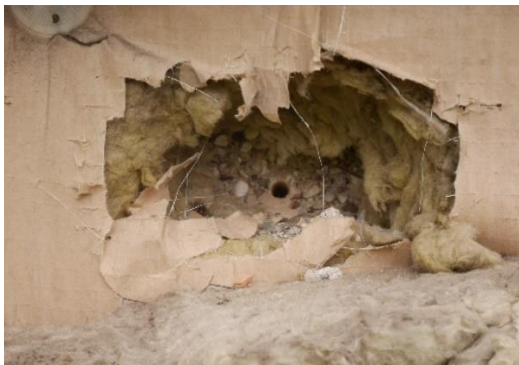
Figure 19. Location 1.4 View showing the original concrete cladding panel with a drilled hole to verify the concrete depth of 100mm without a cavity. Arisings from drilling appeared to be masonry dust only. It would be expected that a layer of EPS insulation has been incorporated within the external wall material although this could not be verified by drilling.
