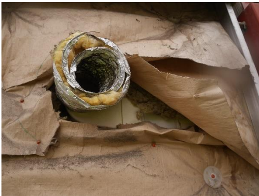
Figure 32. Location 2.2 Kitchen extract tracks horizontally within the insulation depth using a plastic extract duct. The point of entry into the RC structure could not be found and was therefore not surveyed.
