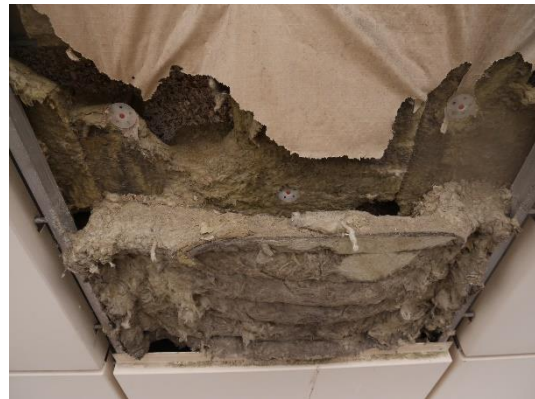
Figure 33. Location 2.2 Cavity barrier shown at first floor level below the kitchen extract. The barrier and insulation above is damaged due to vermin infestation.
