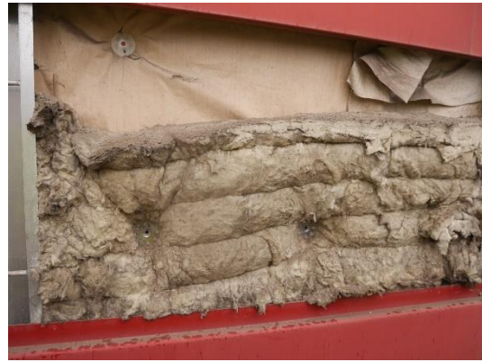
Figure 18. Location 1.4 Horizontal cavity barrier at floor level under window. The vertical aluminium rails offer a pathway through the cavity barriers in the 'u' of the rails. This is however minimal in sectional area.
