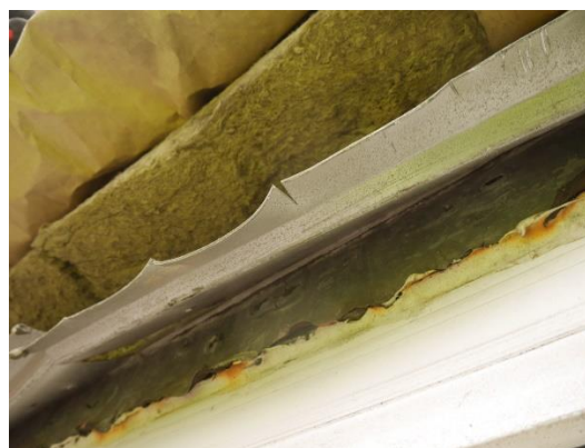
Figure 21. Location 1.5 The mastic seal at the window head appears intact behind the flashing, but is unlikely to be fire resistant.
