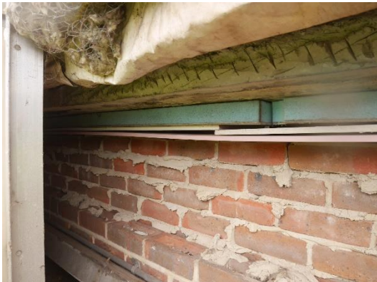
Figure 26. Location 1.7 The first-floor slab is apparent at the top of the image, brickwork infill to the ground floor has been added at a later refurbishment. Vermin droppings are evident on top of the brickwork and top of the metal soffit panel.
