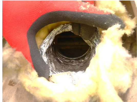
Figure 16. Location 1.3 Ventilation duct passes straight through walling to louvre behind.
