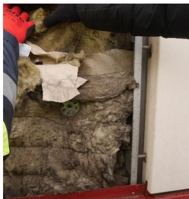
Figure 12. Location 1.1 Gaps identified at side of cavity barrier against cladding support rail, a further gap exists within the insulation behind the rail.
