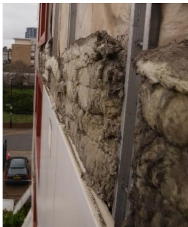
Figure 13. Location 1.2 line of horizontal cavity barrier at floor level, barriers are not folded over and only in partial compression.
