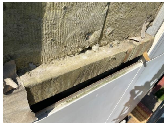
Figure 18. Cavity barrier
