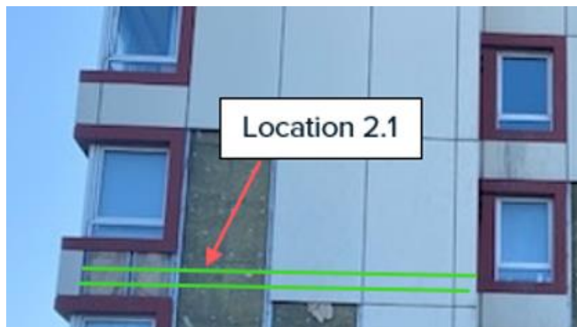
Figure 16. Location 2.1 Missing cavity barrier.
