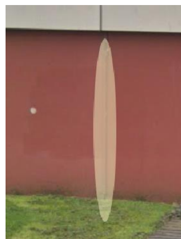
Figure 22. Location 2.4. Close up showing the lightning protection strip
