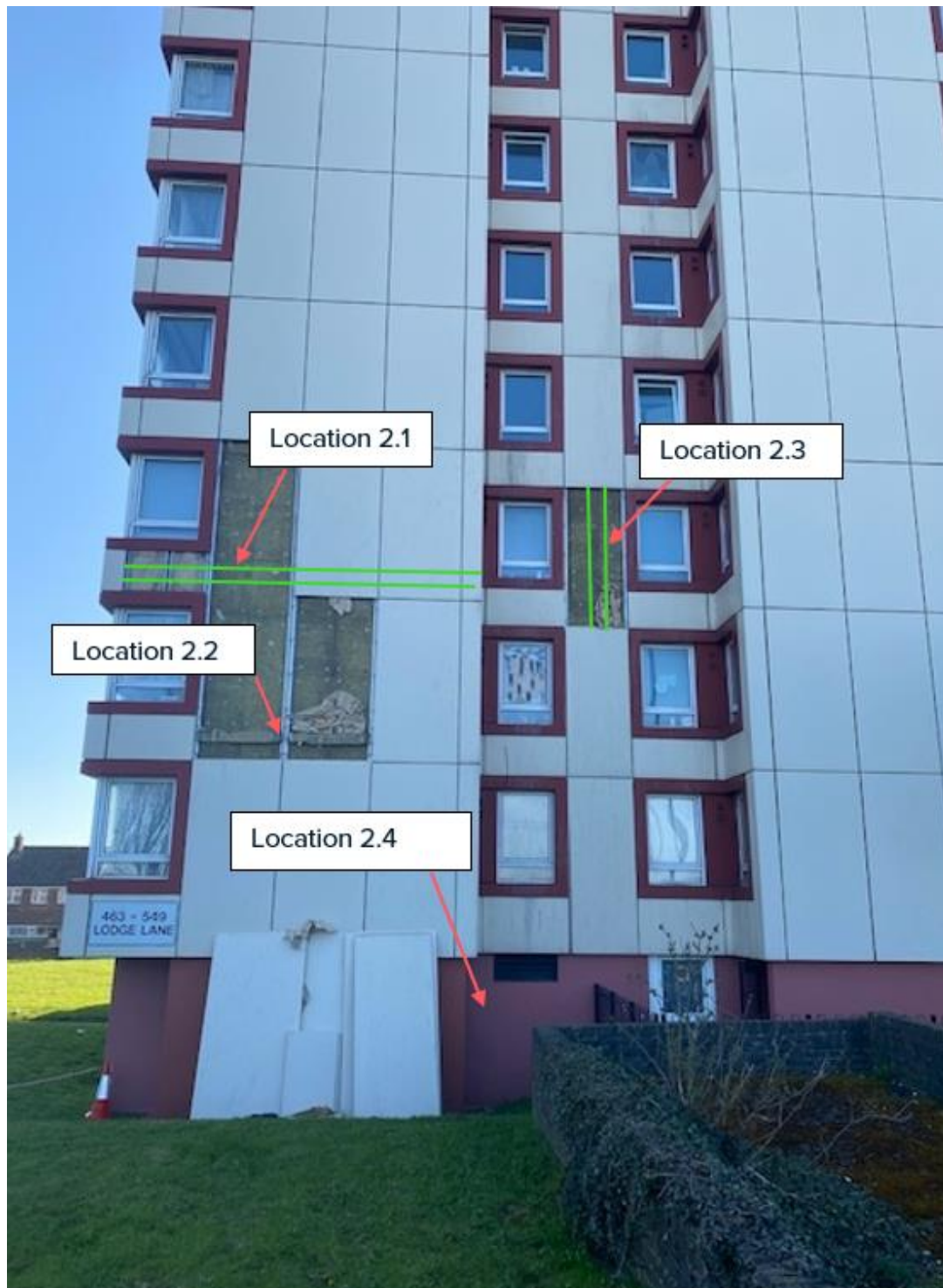
Figure 15. Location 2 areas inspected The green lines indicate internal compartment lines.
