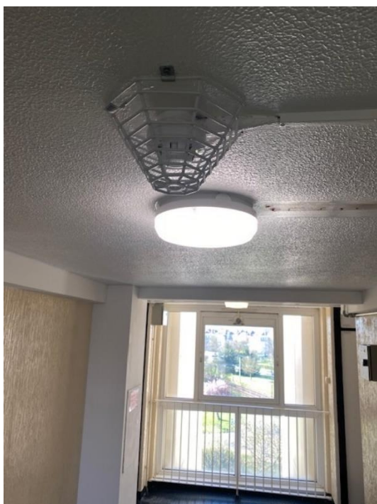
Figure 25. AFD in place to operate the AOV in the lobby
