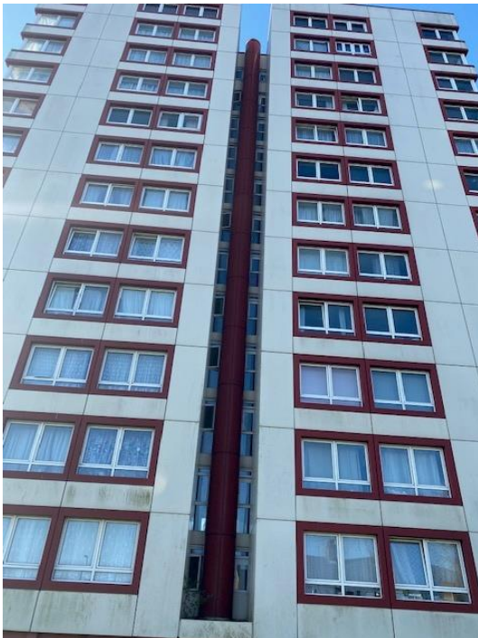
Figure 31. Showing the rubbish chute on the north face of the building
