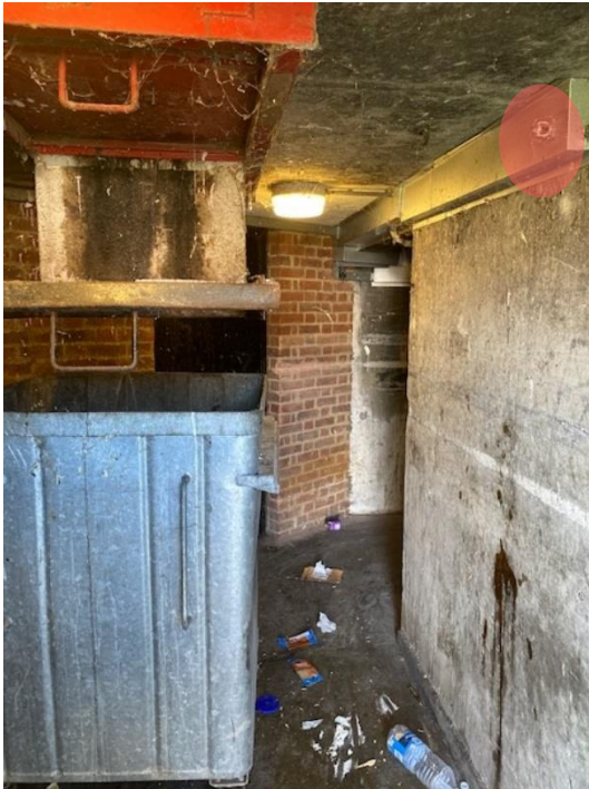
Figure 29. Showing sprinkler head (highlighted) and the spring loaded fire shutter over the wheelie bin
