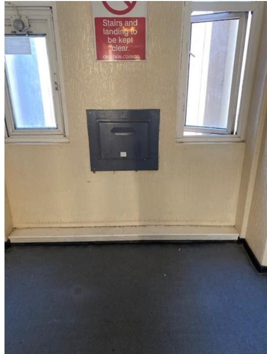
Figure 30. Typical bin chute hopper. An AOV can be seen to the top left.
