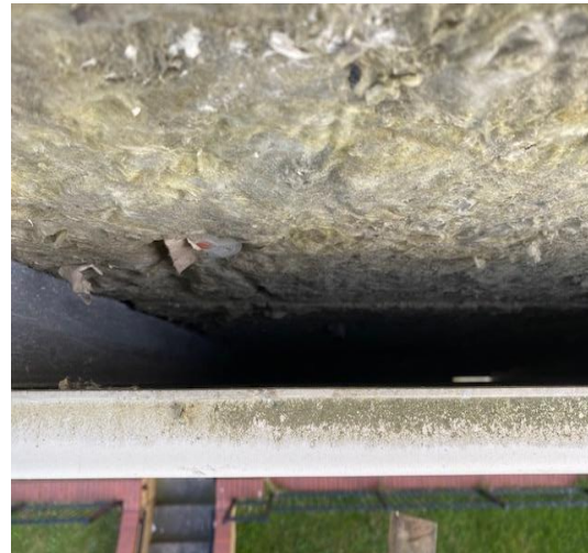
Figure 12. Location 1.1 - Showing the gap between the panelling and insulation, where the cavity barrier should be.
