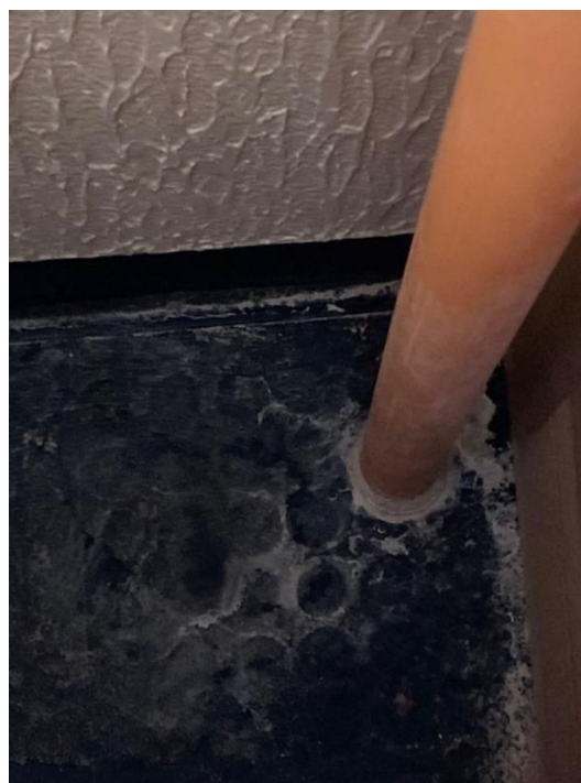
Figure 28. Location 2.4. Close up showing where the sprinkler pipe passes through the compartment floor.
