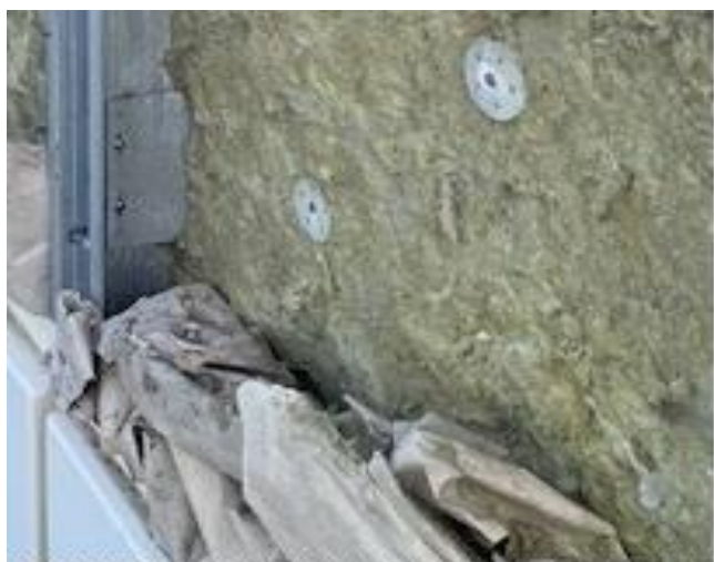
Figure 13. Location 1.2 – Membrane fallen away from the insulation
