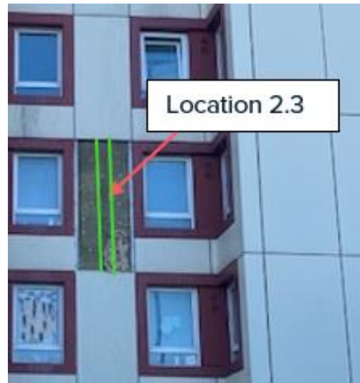
Figure 20. Location 2.3 the equivalent area is shown on the outside of the building. No vertical cavity barrier is in place.
