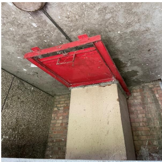
Figure 28. Bin chute damper with fusible link in bin store (example taken from 58-108A Regina Rd)
