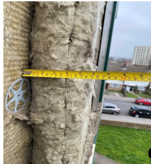
Figure 24. Folded cavity barrier
