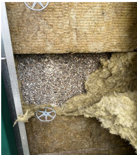
Figure 21. Wall behind mineral wool
