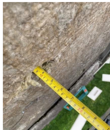
Figure 18. Depth of mineral wool insulation
