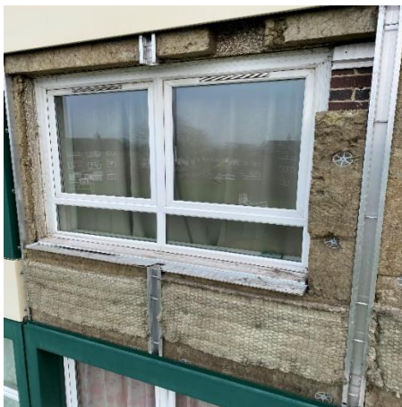
Figure 17. Poorly fitted cavity barrier at compartment floor. Brick wall system can be seen & no cavity barriers around window.
