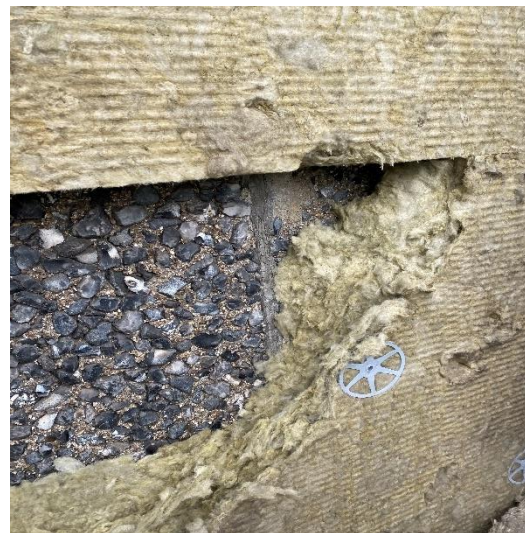
Figure 26. Wall behind mineral wool
