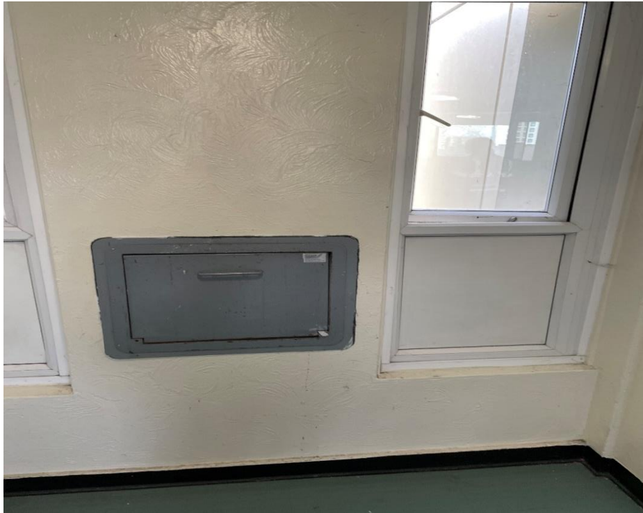
Figure 35. Typical infill panel (taken from 58-108A Regina Rd images)
