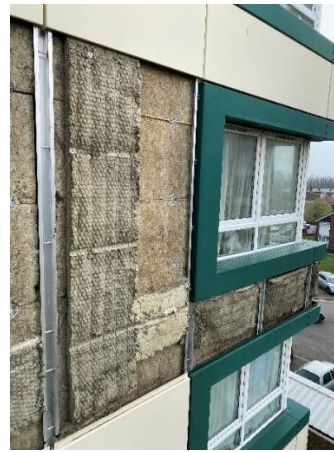
Figure 16. Poorly fitted cavity barriers around window
