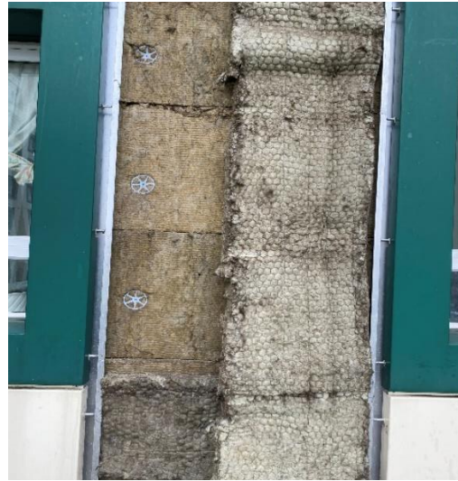
Figure 20. Vertical compartment line not under compression.
