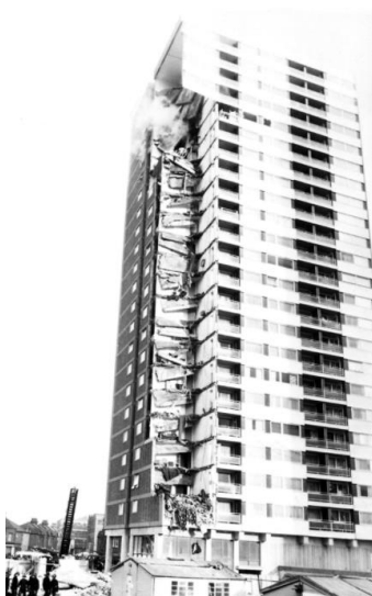
Figure 5. Ronan point collapse
