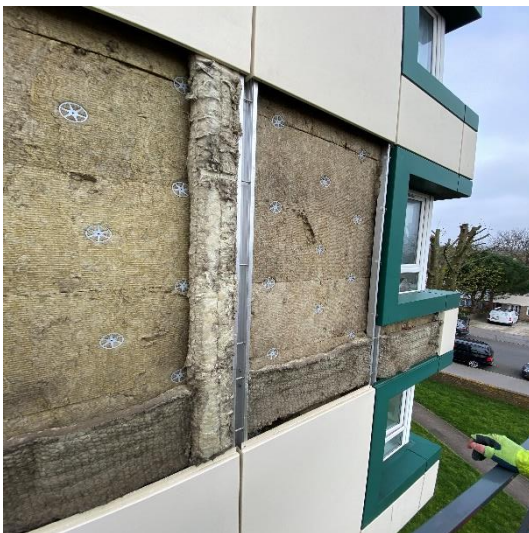
Figure 25. Non folded horizontal barrier
