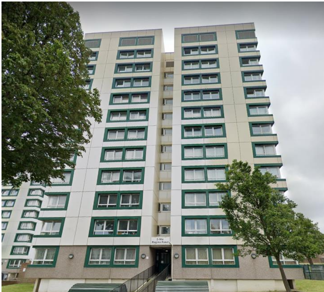
Figure 27. Infill panels
