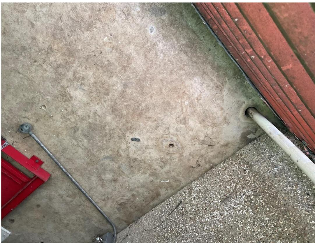
**Figure 32.** Location 5 penetrations in bin store roof – the RC roof has fresh air above.
