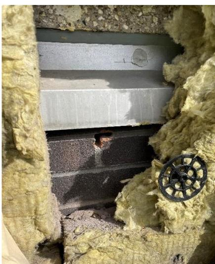
**Figure 28.** Location 4 Junction between the brickworks and concrete LPS panels exposed. Metal rain drip tray in position
