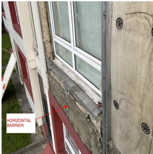
**Figure 20.** Location 1.3 horizontal cavity barrier
