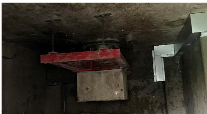
**Figure 35.** Bin store fusible link and sprinkler
