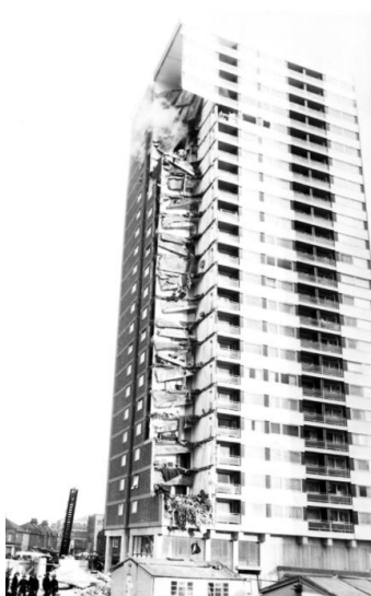
Figure 5. Ronan point collapse
