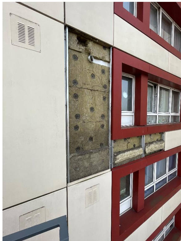
Figure 15. View of barrier not folded on the continuous cladding section, however the barrier has been folded at the area between openings.
