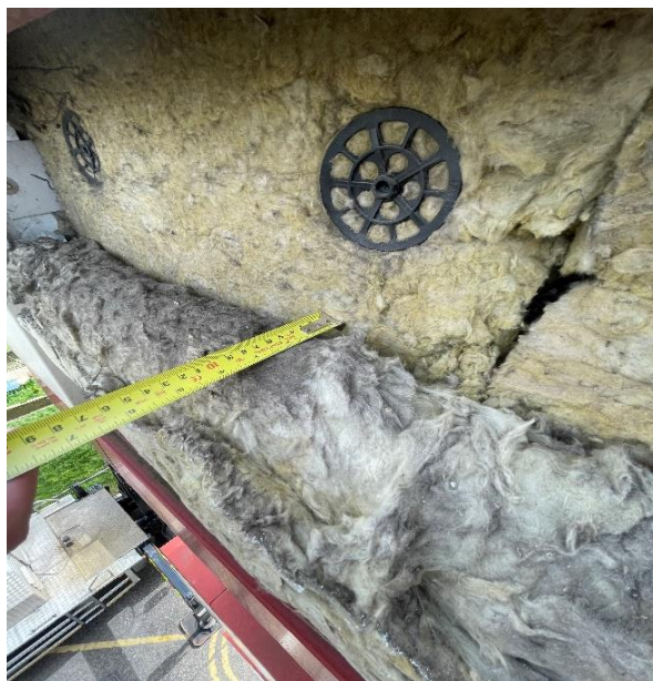
Figure 16. View behind metal cladding Figure 17. Measurement of barrier
