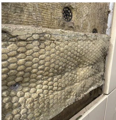
Figure 23. Barrier incorrectly installed
