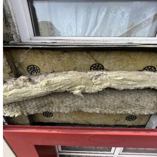
Figure 27. Poorly fitted cavity barrier under window
