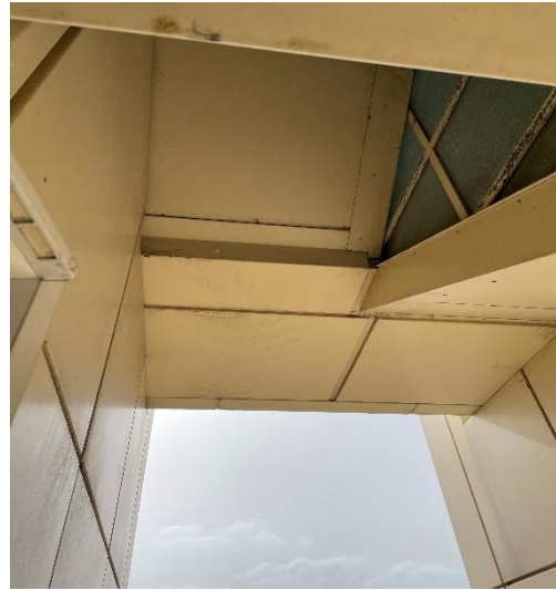
Figure 34. Overhang from inside block with Georgian wire glass
