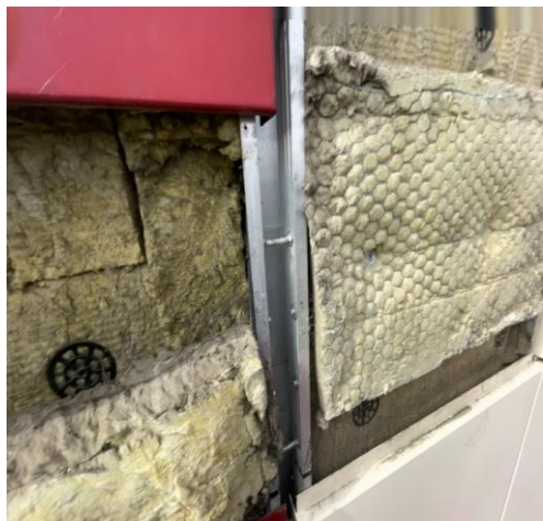
Figure 21. Cavity barrier not folded next to correctly installed barrier
