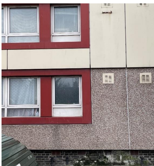
Figure 12. View of location of render with PIR cladding system behind
