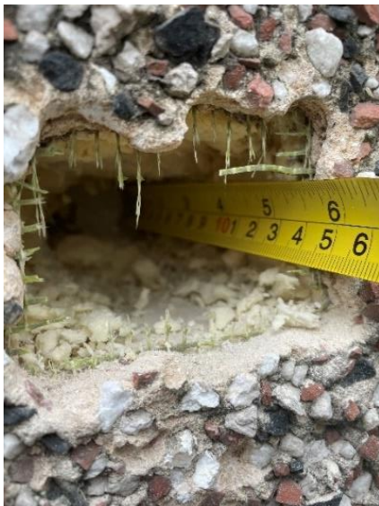
Figure 24. Location 2.1 – 150mm deep insulation to concrete behind
