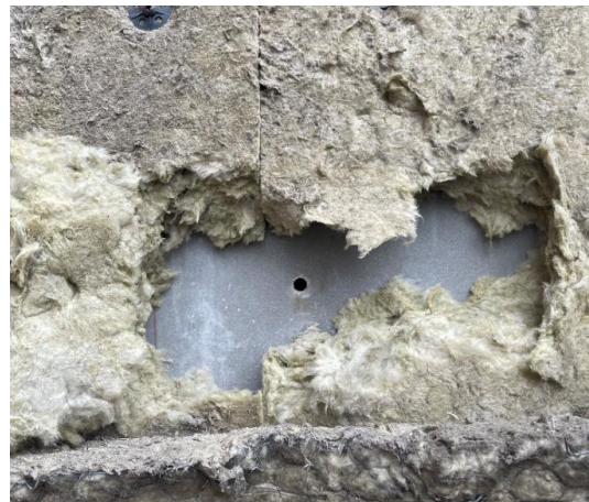
Figure 36. Location 4 approx. 10mm thick CPB
