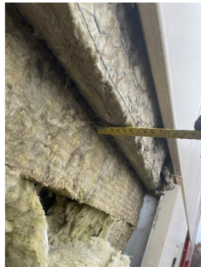
Figure 15. Location 1.2 70mm cavity barrier at 3 rd floor level.
