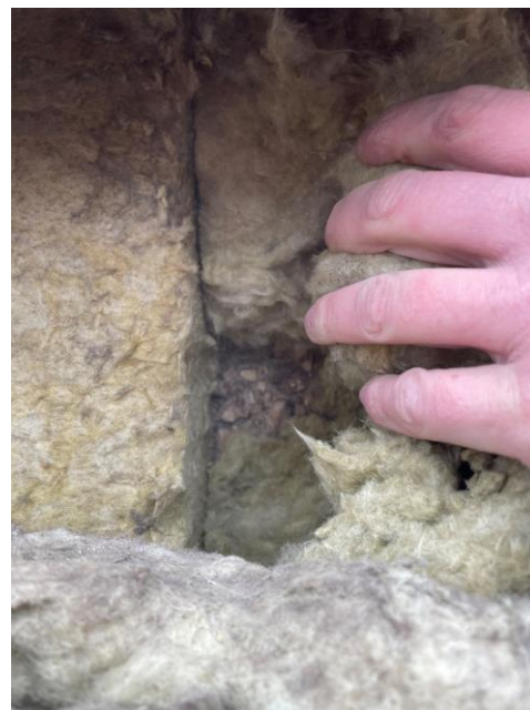
Figure 30. Location 3.1 solid concrete behind 100mm mineral wool insulation
