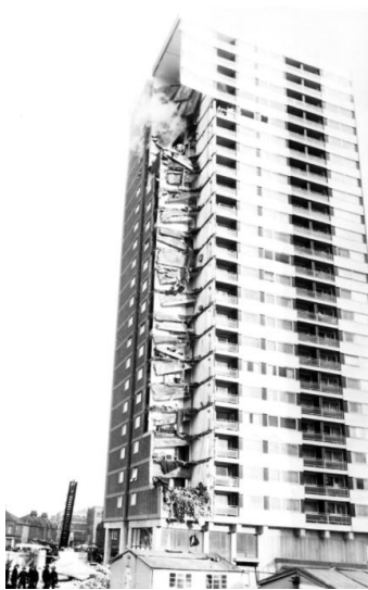
Figure 4. Ronan point collapse
