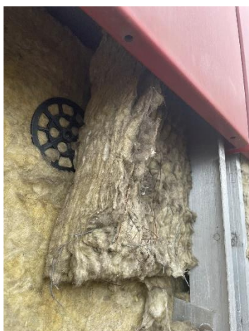
Figure 19. Location 1.4 vertical cavity barrier damaged and not under compression
