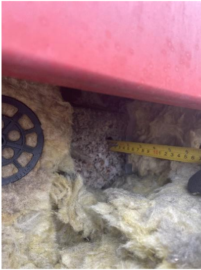
Figure 12. Location 1.1 solid concrete behind 100mm mineral wool insulation
