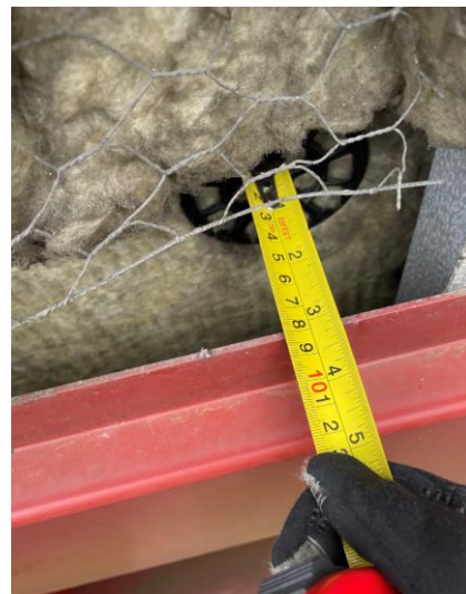
Figure 33. Location 3.3 80mm cavity between insulation and panel
