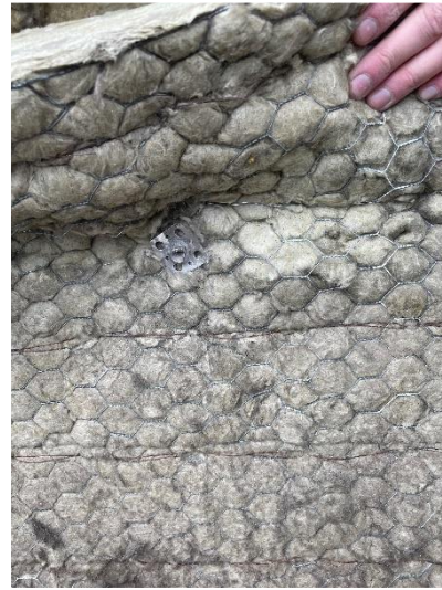
Figure 13. Location 1.1 cavity barrier with robust metal fixing and reinforced with mineral wool
