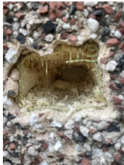
Figure 25. Location 2.1 - 3-5mm of render with thermo plastic insulation behind
