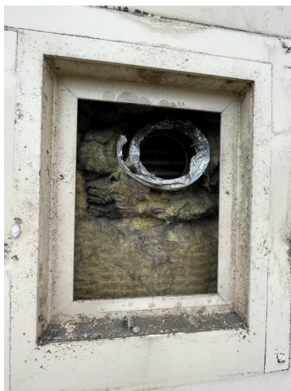
Figure 21. Location 1.5 kitchen extract with no cavity barrier
