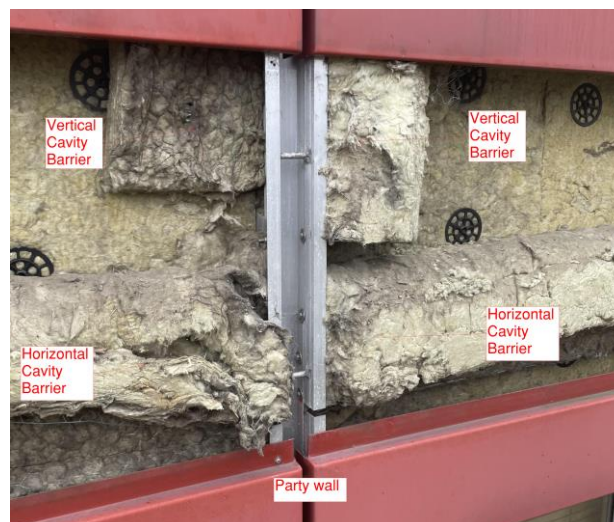
Figure 18. Location 1.4 horizontal and vertical cavity barriers identified.
