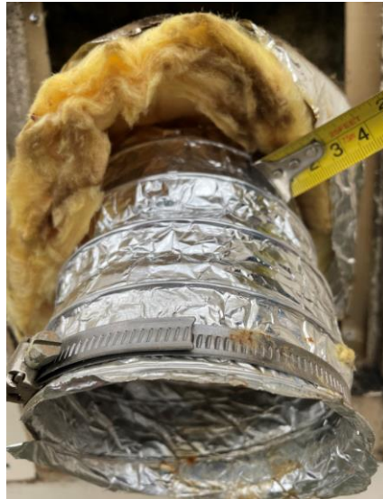
Figure 31. Location 3.2 duct to outside wrapped in 30mm mineral wool
