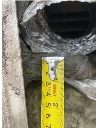
Figure 17. Location 1.3 30mm mineral wool encapsulating ductwork
