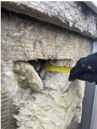
Figure 14. Location 1.2 concrete behind 100mm mineral wool
