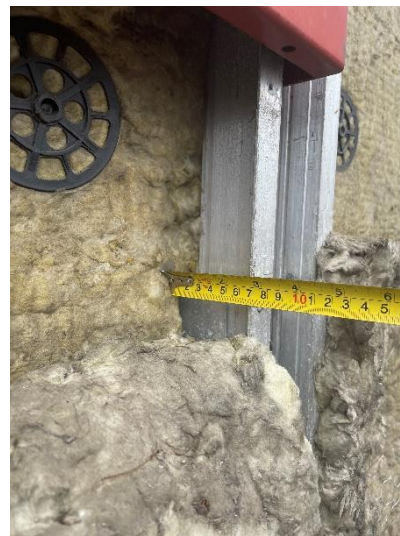
Figure 11. Location 1.1 70mm clear cavity
