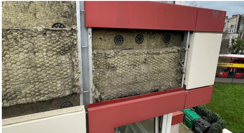
Figure 22. Location 1.6 horizontal cavity barrier not continuous or folded over
