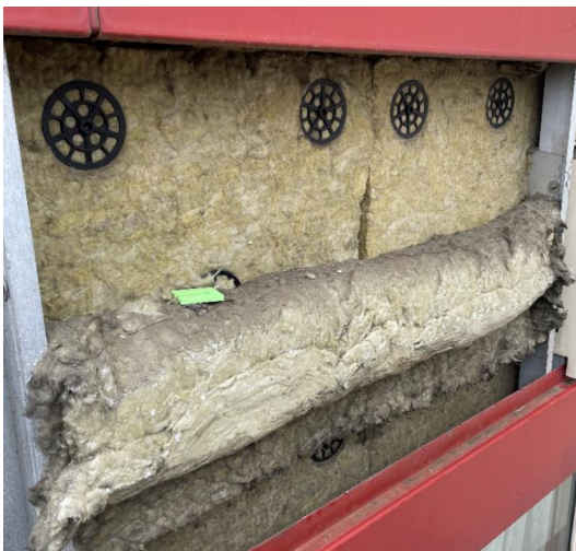
Figure 32. Location 3.3 horizontal cavity barrier
