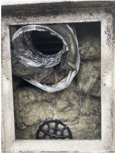
Figure 16. Location 1.3 kitchen extract ductwork wrapped with mineral wool
