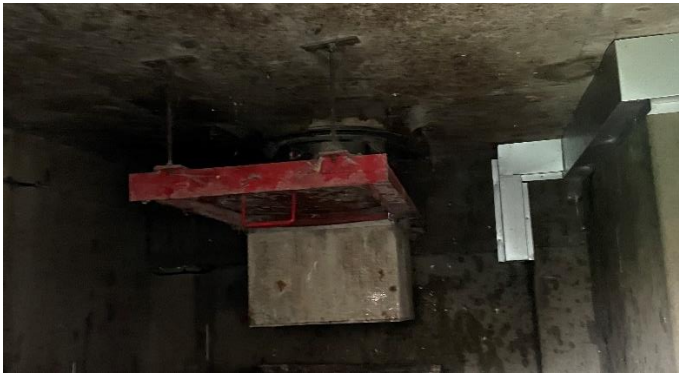
Figure 38. Bin store fusible link and sprinkler
