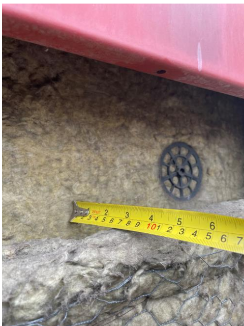
Figure 29. Location 3.1 100mm horizontal cavity barrier on top of mineral wool insulation
