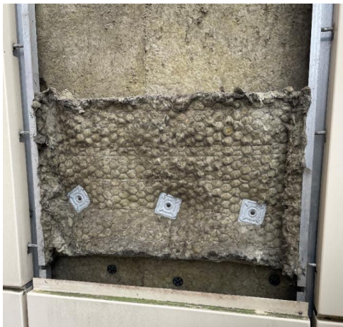
Figure 35. Location 4 horizontal cavity barrier mechanically fixed but not folded over
