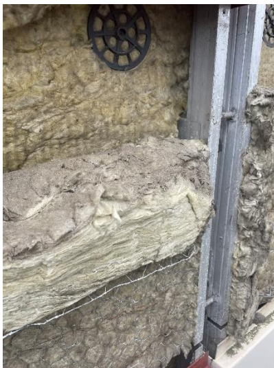
Figure 10. Location 1.1 horizontal cavity barrier folded over and under compression
