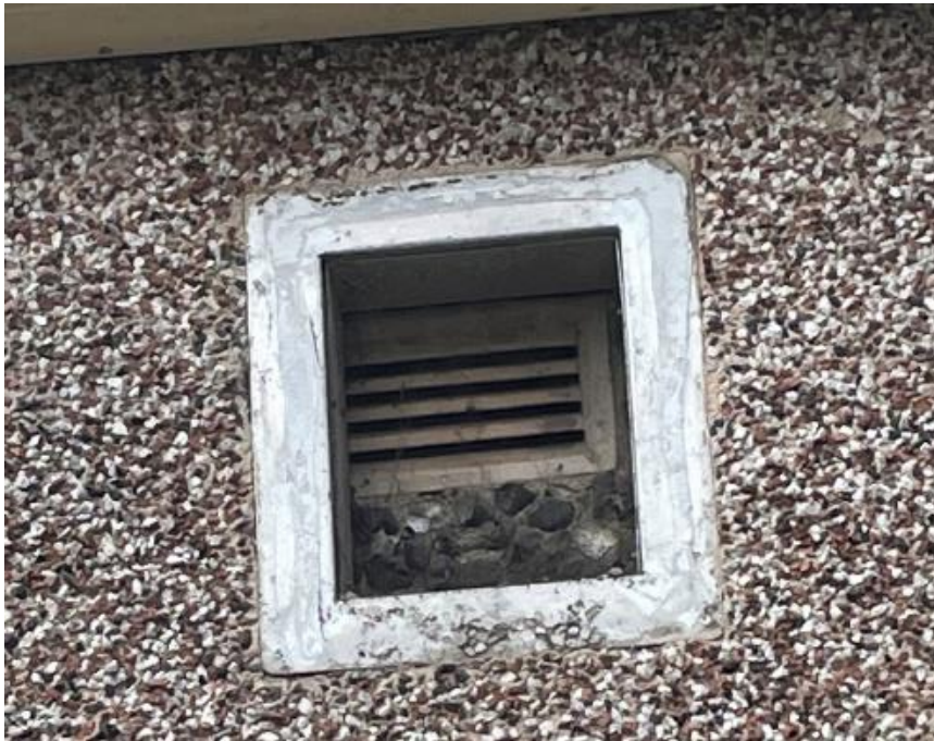
Figure 27. Location 2.2 extract boxed in with steel
