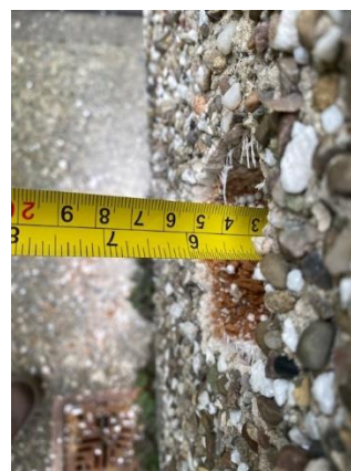
Figure 20. Location 2.1 - 3-5mm of render with 145mm of insulating material
