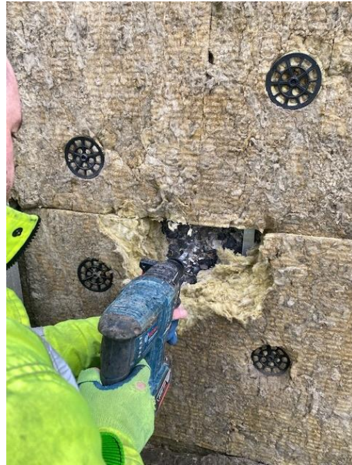
Figure 13. Location 1.2 cavity barrier with robust metal fixing and reinforced with mineral wool
