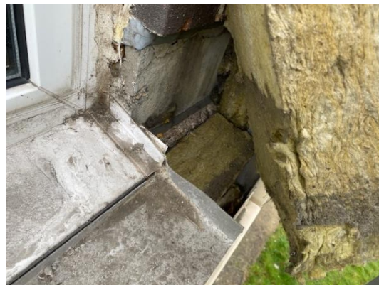
Figure 11. Location 1.1 Showing that there are no cavity barriers in place around the window openings. Original building features can be seen.
