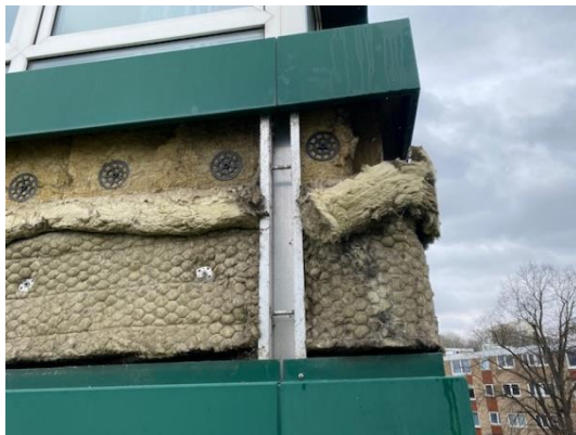
Figure 10. Location 1.1 horizontal cavity barrier folded over and under compression
