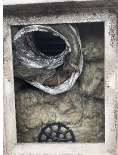
Figure 15. Location 1.3 30mm mineral wool encapsulating ductwork
