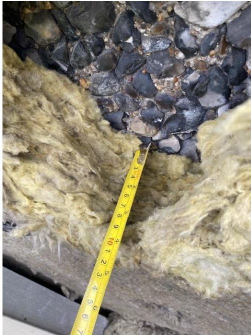
Figure 12. Location 1.2 solid concrete behind 100mm mineral wool insulation
