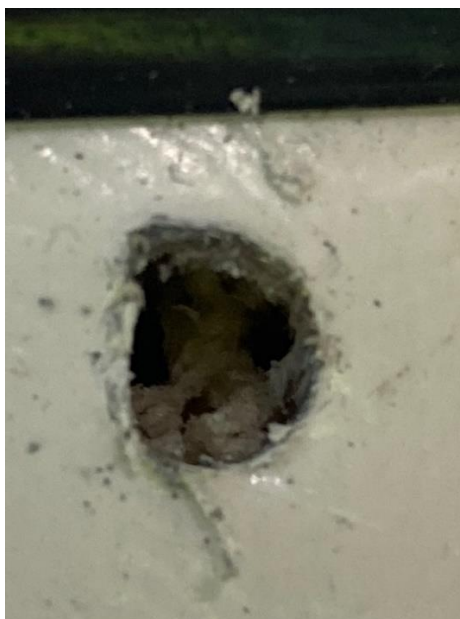
Figure 23. Infill panel showing the infill material between the steel
