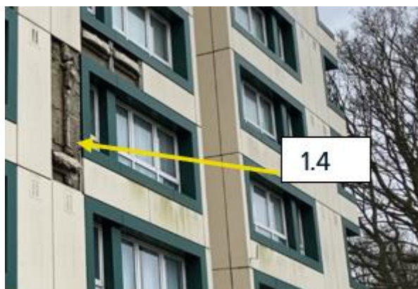
Figure 16. Location 1.4 horizontal and vertical cavity barriers identified.
