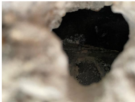
Figure 38. Location 4.4 close-up of the drill hole through the stone cladding system
