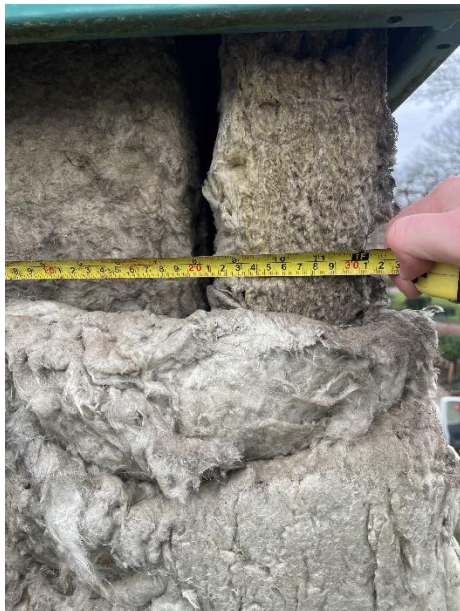
Figure 15. Location 2.1 horizontal cavity barrier around the corner
