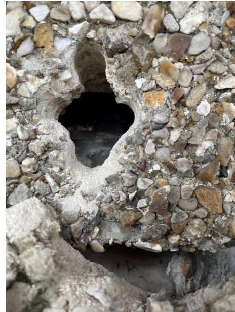
Figure 37. Location 4.4 drill hole through the stone cladding system
