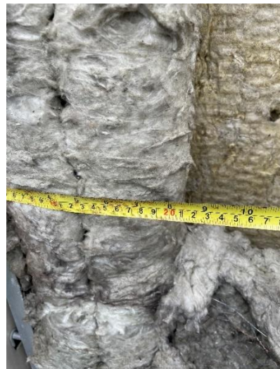
Figure 33. Location 4.2 junction of horizontal and vertical cavity barriers
