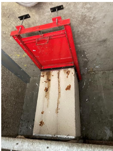
Figure 43. Bin chute fusible link
