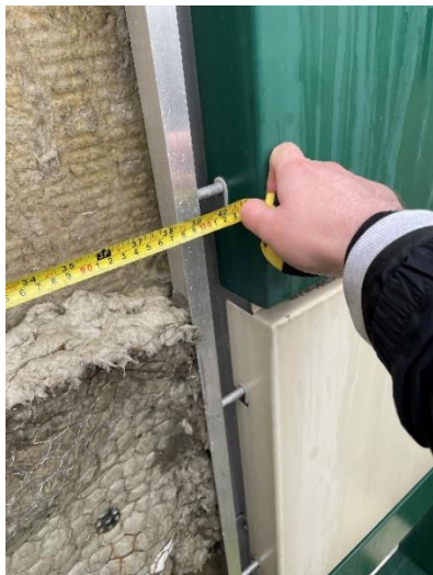
Figure 32. Location 4.2 / 4.3 horizontal cavity barrier at slab level only. There is no vertical cavity barrier around the right hand window.
