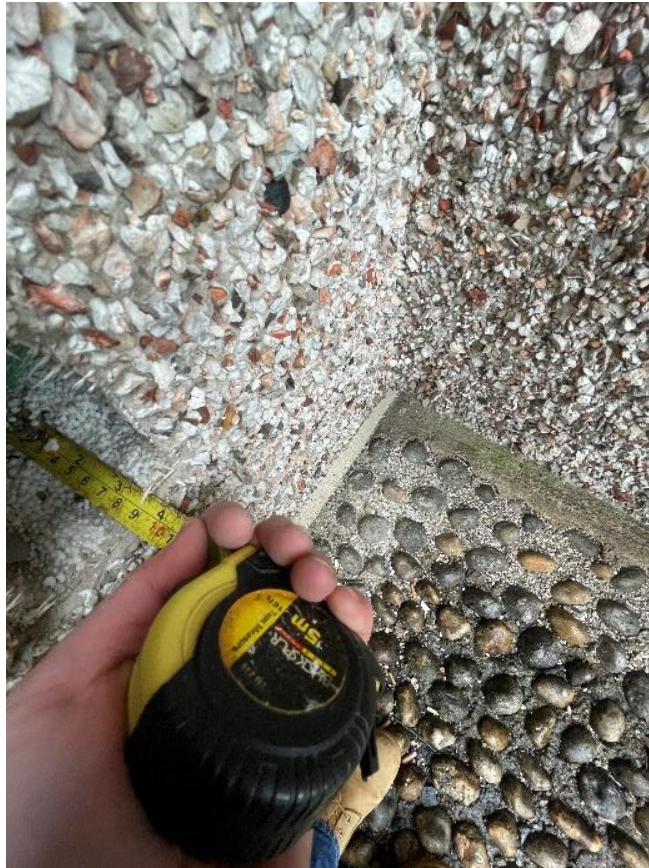
Figure 28. Location 3 shows 90mm depth of EPS system at ground floor
