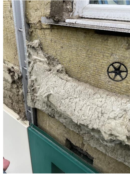
Figure 22. Location 2.3 folded horizontal cavity barrier approximately below the window. Letterbox of removed insulation
