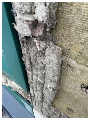
Figure 19. Location 2.2 vertical cavity barrier around the window
