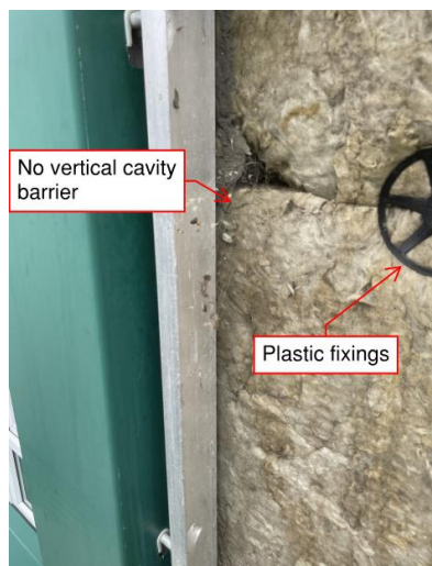
Figure 10. Location 1.1 no vertical cavity barrier
