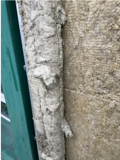
Figure 30. Location 4.1 vertical cavity barrier around window and between two flats
