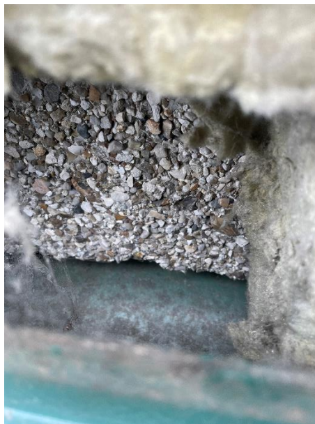
Figure 23. Location 2.3 original rough stone concrete behind the insulation
