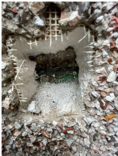
Figure 26. Location 3 EPS behind stone cladding system. The original RC structure can be seen at the rear of the cavity
