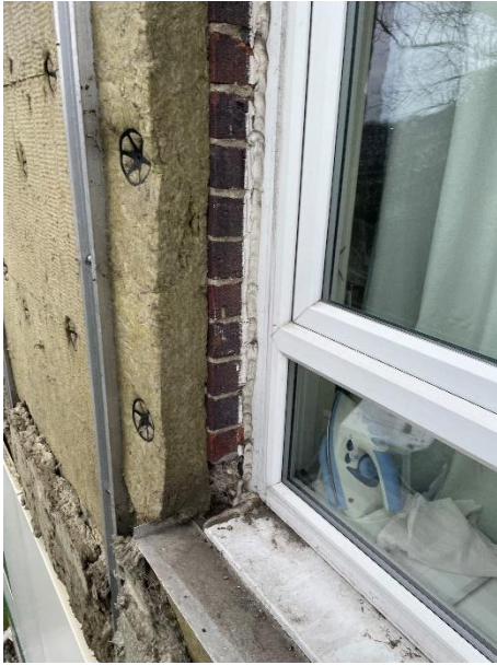
Figure 21. Location 2.3 exposed brick and mastic surrounding the window frame
