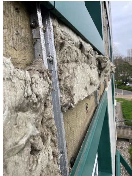
Figure 16. Location 2.1 horizontal cavity barrier is not continuous due to the aluminium rails and changes level under the window
