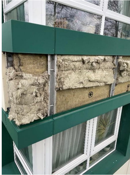
Figure 17. Location 2.2 cavity barriers are not continuous below the window or at slab level
