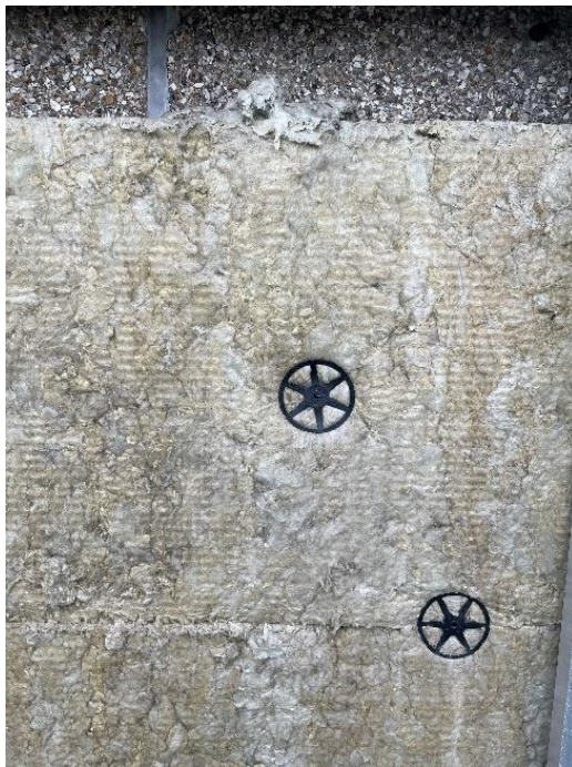
Figure 34. Location 4.4 where the cavity is not fully filled with insulation
