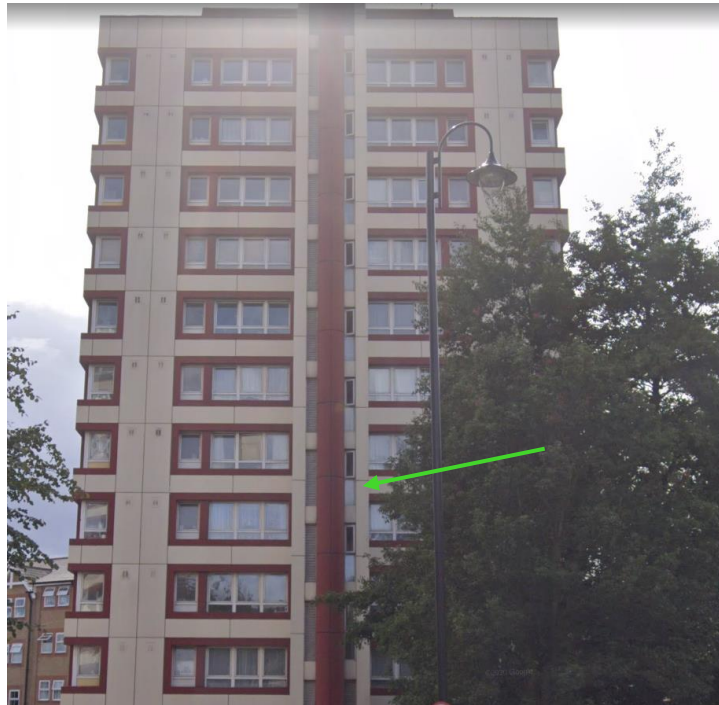
Figure 43. Infill panels
