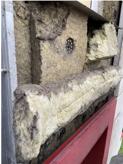
Figure 15. Location 1.3 horizontal cavity barrier folded over and under compression
