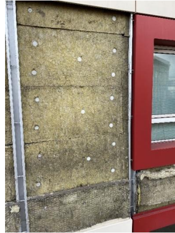
Figure 40. Location 3.3 no vertical cavity barriers around window
