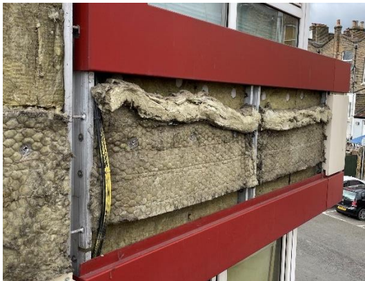
Figure 41. Location 3.4 horizontal cavity barrier broken due to aluminium rail. Wires also identified in the cavity.
