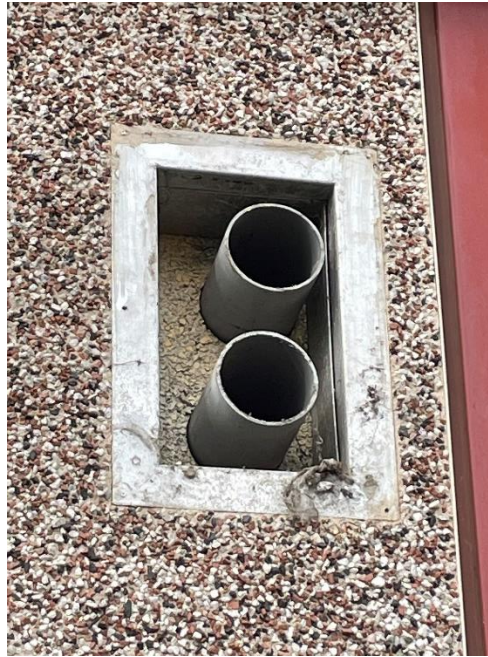
Figure 30. Location 2.2 ductwork enclosed in 'letterbox'
