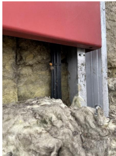
Figure 36. Location 3.1 wires were identified within the cavity.
