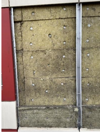
Figure 39. Location 3.3 mineral wool insulation with horizontal cavity barrier at floor level (not folded over)
