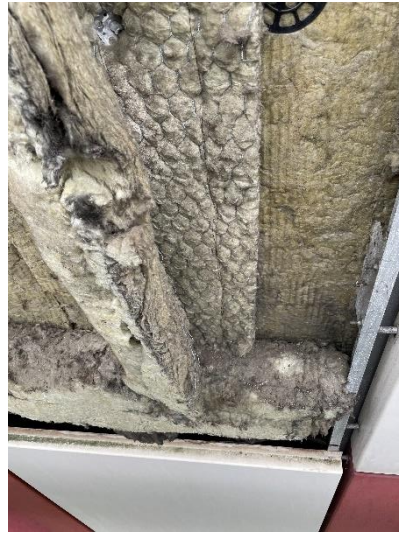
Figure 20. Location 1.4 horizontal cavity barrier at floor level. Not continuous due to aluminium rail.
