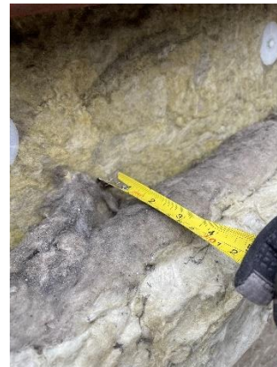
Figure 42. Location 3.4 100mm cavity barrier partially folded at the top
