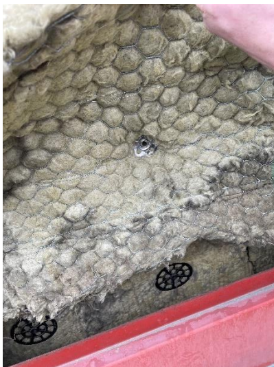
Figure 17. Location 1.3 cavity barrier reinforced with wire and provided with metal fixings to the structure behind
