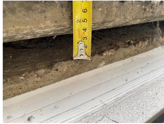
Figure 13. Location 1.2 40mm gap between LPS and infill panel
