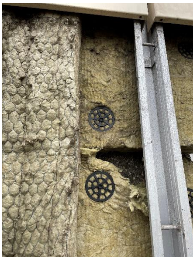
Figure 10. Location 1.1 vertical cavity barrier reinforced with wire but not folded over
