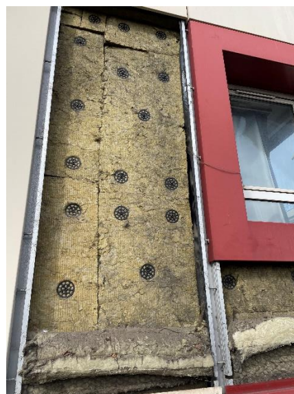
Figure 25. Location 1.6 horizontal cavity barrier at floor level identified but no vertical around the window
