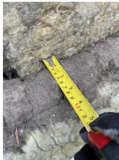
Figure 18. Location 1.3 100mm cavity barrier folded over and under compression
