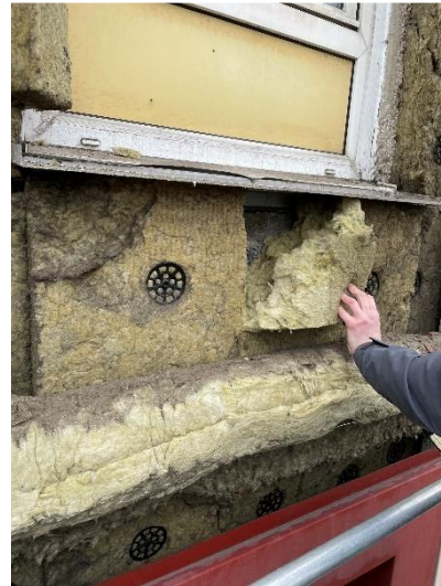
Figure 16. Location 1.3 original window frame behind insulation
