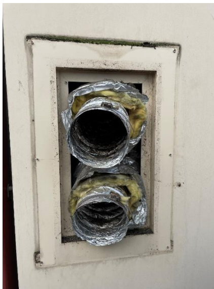
Figure 23. Location 1.5 Mineral wool wrapped around the ductwork from second floor flat
