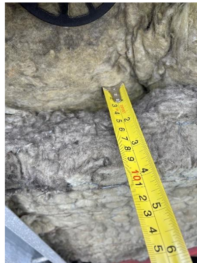
Figure 34. Location 3.1 70mm cavity barrier on top of mineral wool insulation
