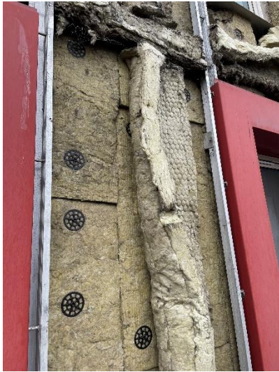
Figure 19. Location 1.4 vertical cavity barrier on top of insulation
