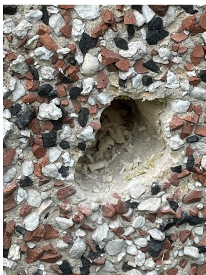
Figure 27. Location 2.1 3-5mm of render with thermo plastic insulation behind
