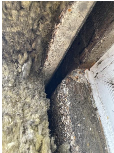
Figure 14. Location 1.2 concrete infill panel above window with 40mm gap
