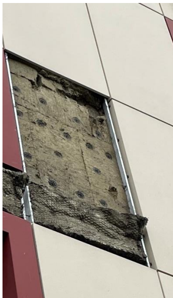
Figure 37. Location 3.2 there was no vertical cavity barrier identified
