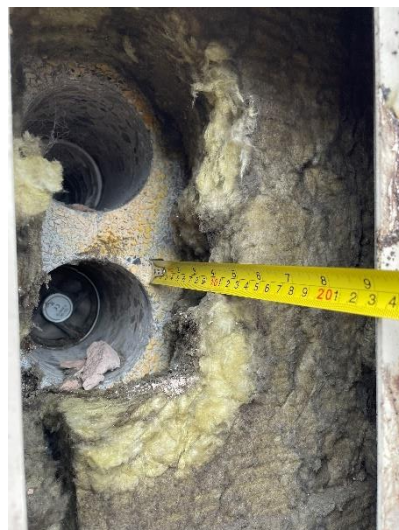
Figure 22. Location 1.5 no cavity barrier
