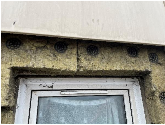
Figure 12. Location 1.2 no cavity barrier around window
