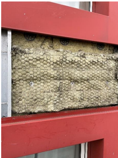
Figure 33. Location 3.1 horizontal cavity barrier reinforced with wire but not folded over
