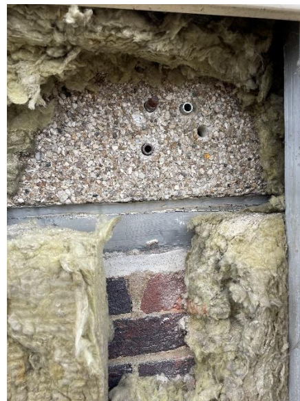
Figure 38. Location 3.2 masonry construction behind mineral wool insulation
