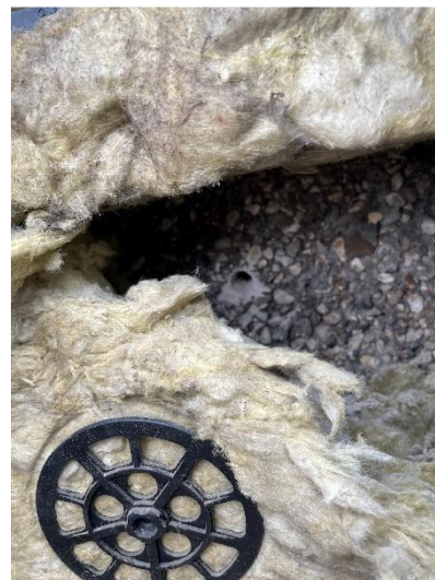
Figure 11. Location 1.1 cavity between solid concrete and aluminium panel
