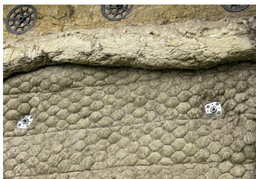
Figure 10. Location 1.1 horizontal cavity barrier with mechanical fixings.
