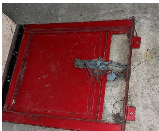
Figure 26. Bin store automatic shutter – fixed open with rope.
