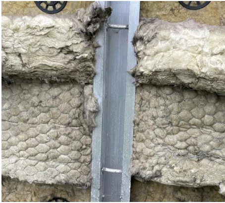
Figure 20. Location 3.1 - 100mm break in cavity barrier for an aluminium bracket.
