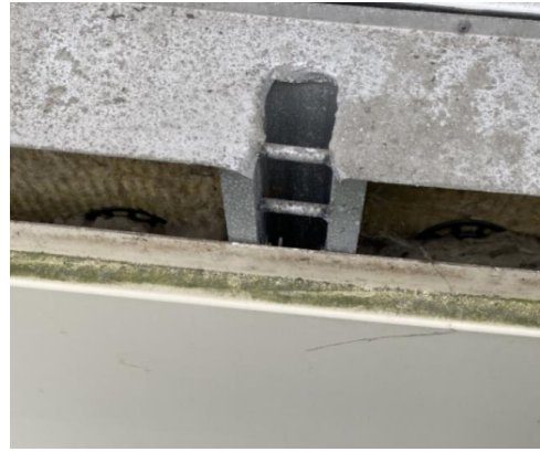
Figure 21. Location 3.3 - 100mm break in cavity barrier for an aluminium bracket. This bracket is hidden behind wider cladding panels, providing an additional fixing point for the panels.
