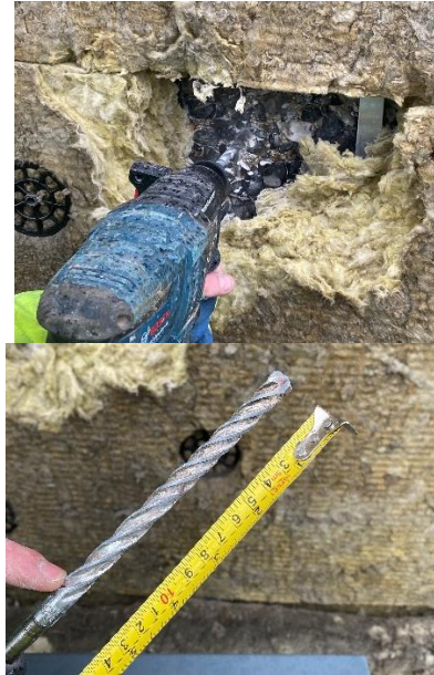
Figure 19. Location 3.2 - 100mm hole drilled in concrete
