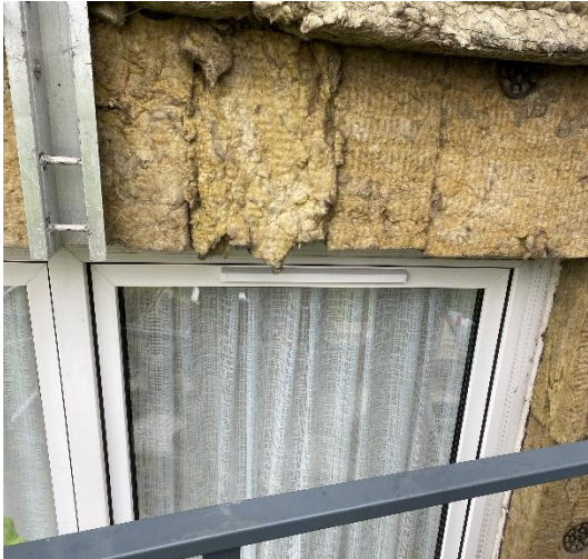
Figure 16. Location 3.1 – no cavity barriers provided around window openings.
