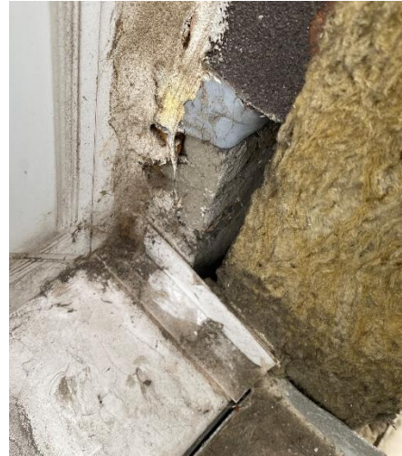
Figure 17. Location 3.1 – grey silicon/rubber expansion joint between the concrete compartment floor and the LPS panels.
