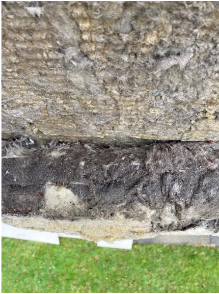
Figure 18. Location 3.2 folded cavity barrier.
