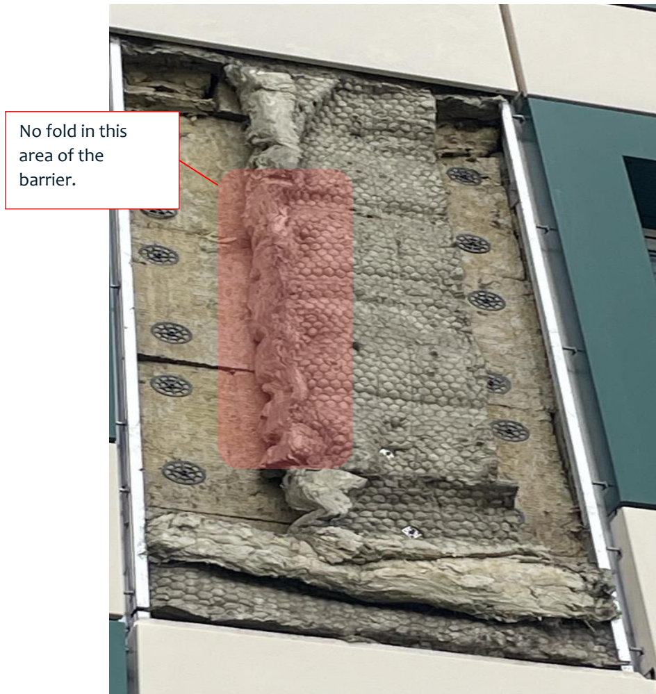
Figure 23. Location 4 – The vertical cavity barrier is not folded in the area highlighted.
