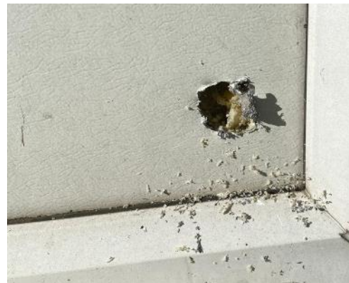
Figure 25. Location 5 – hole drilled and an unknown thermoplastic identified within the panel.
