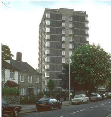
Figure 1. 1-44 Bramley Hill, showing original external 'LPS' walls, photo circa 1985.
