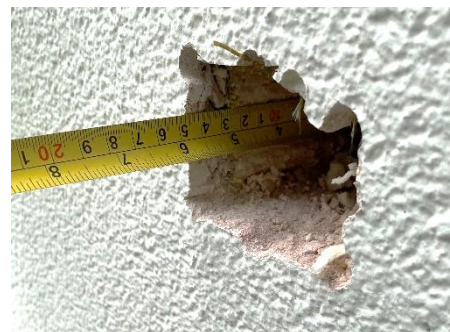
Figure 14. Location 2 – Polyurethane foam and measurement.
